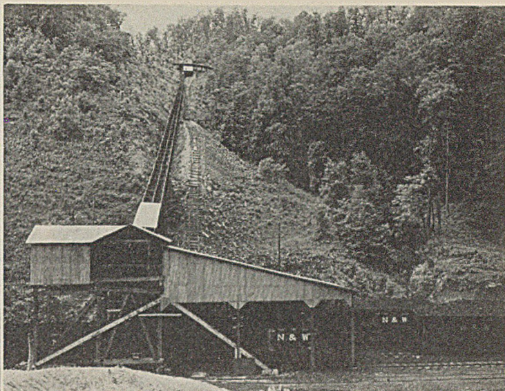
Home Creek Smokeless Coal Co. Plant and Retarding Rope-and-Button Conveyor. This Operation Shipped the First Coal From the Grundy Field
