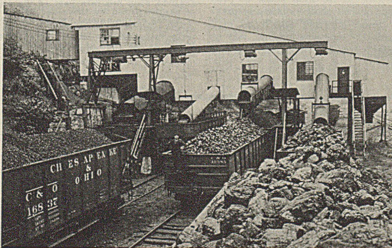
Coal From the Saw Section Improves the Appearance of the Lump Output From the Whole Mine.
