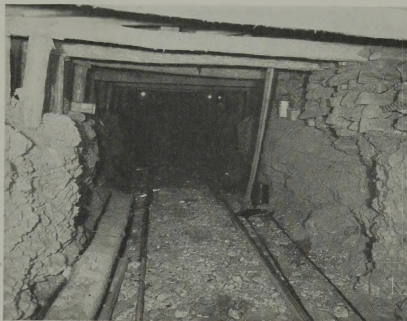
Fig. 4—View of Roadway Ahead of Wall Showing Timbering and Hoist Tail Block.
