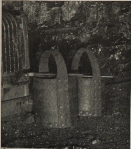
These Leather Boxes Reduce Bit Loss at Knox Consolidated Mines.
