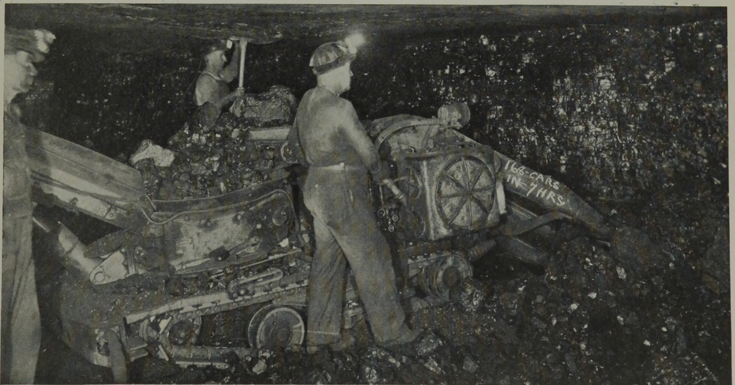
Fig. 1—Loading Cut in a 30-ft. Place.
