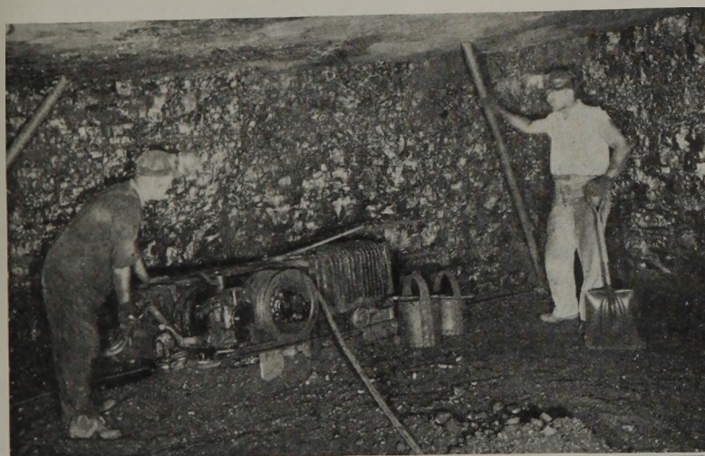
Fig. 4—Portable Transformer Unit Employed at Knox Consolidated Mines.
