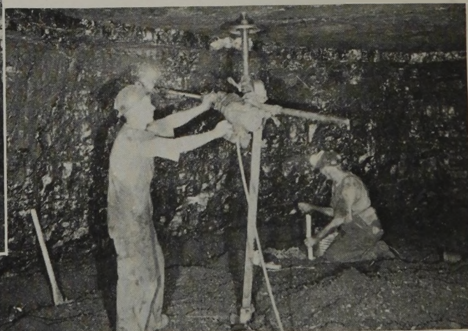
Fig. 3—Drilling Crew at Work in a Wide Place.
