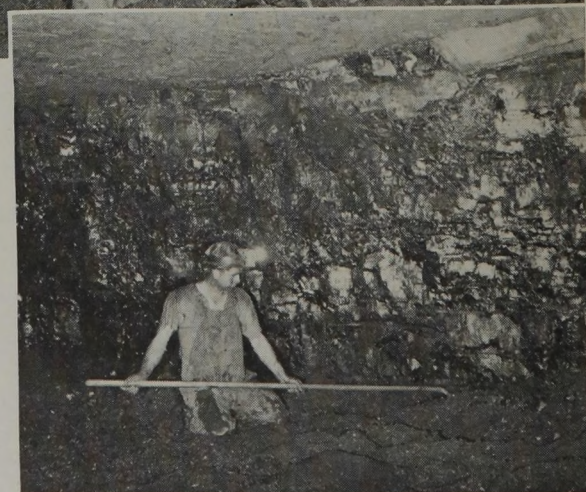
Fig. 5—Bug-Dusting in Preparation for Snubbing on the Night Shift.
