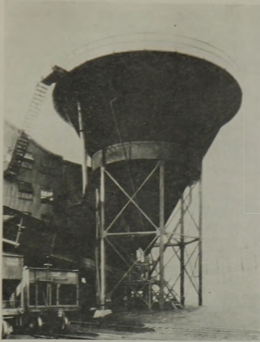
Settling Tank From Which Overflow Goes to Jigs.
