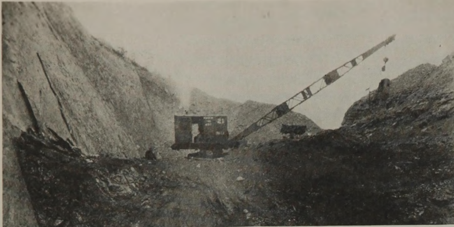
Fig. 2—Stripping at Maryd Colliery Showing Coal Being Removed From a Sharp Fold by a Dragline Working Along the Length of the Pit.
