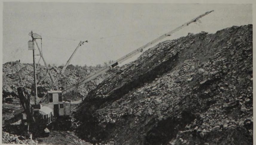
Fig. 1—Huntsville Car Transporter. Spoil Is Elevated to Top of Bank by a Car Running on the Inclined Bridge. Dumping Is Automatic.
