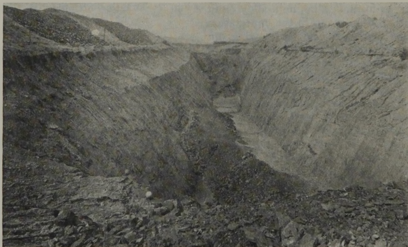
Fig. 3—Richards Stripping. Coal Has Been Removed at Near End and Is Now Being Mined in Rear. Shows Present Road Into Stripping and Dividing Rock in Seam Being Dumped at Near End to Make New Road.
