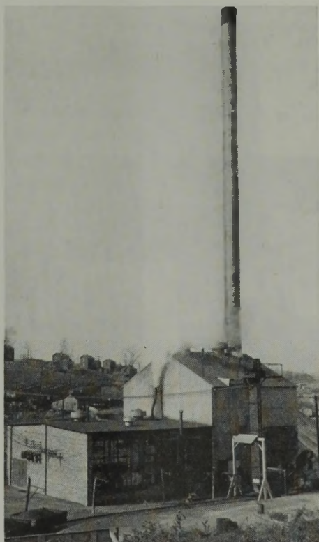
Car-Hoist Frame, Coal Elevator and Inclined Cinder Conveyor Are to Be Seen on the Near Side of the Boiler House.
