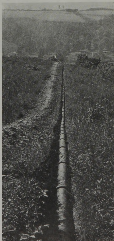
Six-Inch Cast-Iron Pipe From Filter Plant to Storage Tanks.
