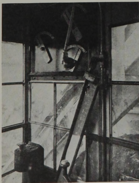
Fig. 4 — Above, Caterpillar Position Indicators; Below, Indicator Showing Position of Car on Bridge.
