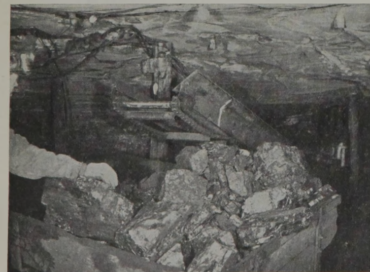
Loading Stations Are Made by Blasting Down Top to Accommodate the Loading Head.
