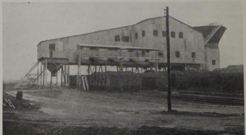
Delta Preparation Plant From the Loading-Boom Side.
