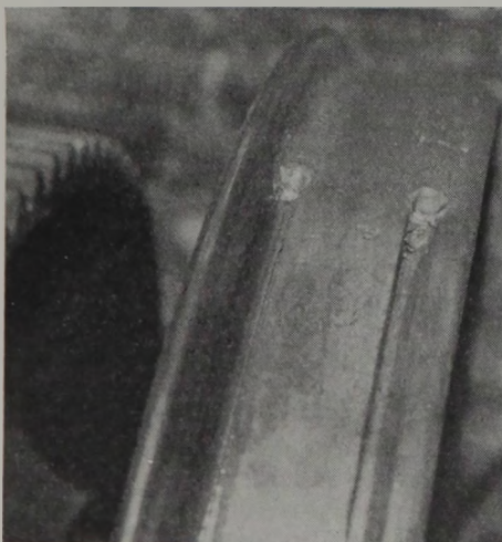
Band Welding Partially Completed.
