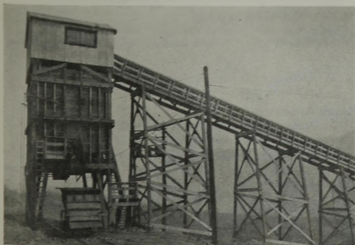
The Larry Travel From Refuse Bin to Dump Is but a Few Hundred Feet.
