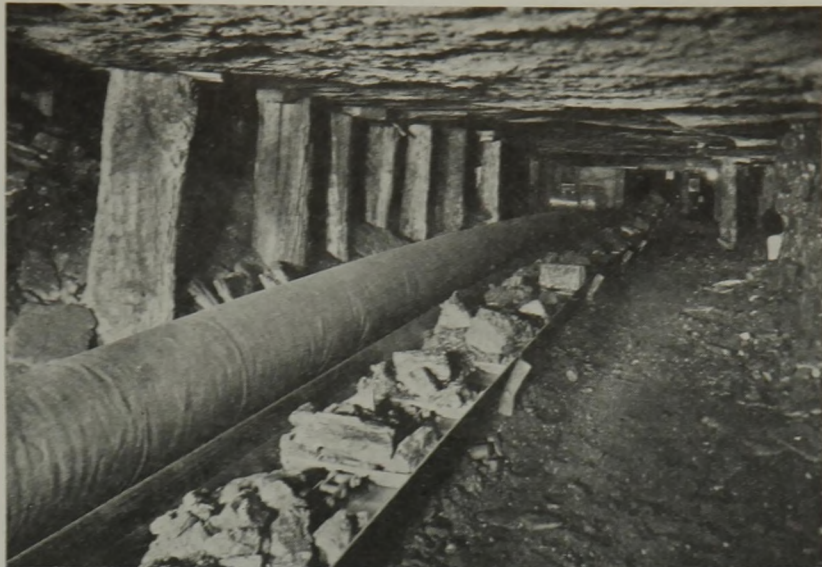
Ventilation Tube and Room Conveyor. The Mother Belt Conveyor Is Installed in the Heading Just Back of the Blower.
