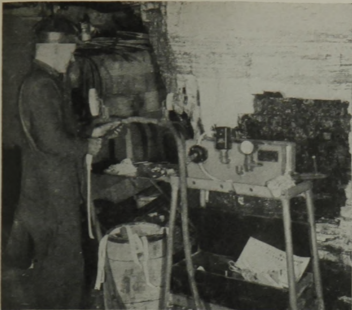
For Safety and Efficiency, Trailing Cables Are Spliced and Vulcanized.
