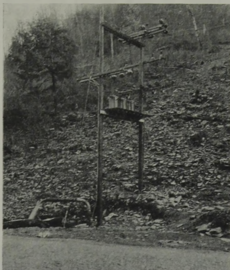
Installation at the Top of the Borehole.
