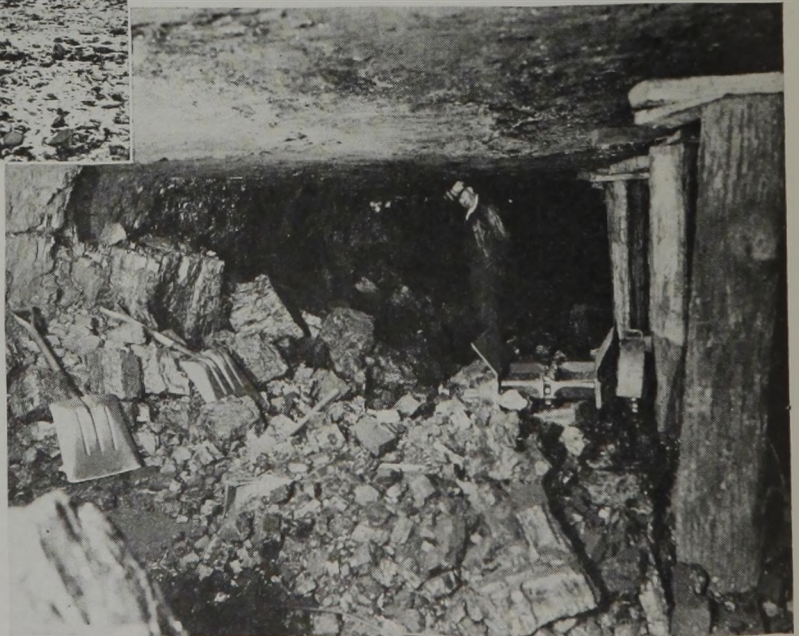
Face Conveyor in No. 5 Mine. With Speedy Working, the Top Holds Nicely.
