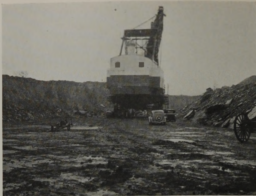
Overburden Is Removed by a 10-Cu.Yd. Stripping Shovel After Being Drilled With the Horizontal Drill Shown in the Foreground and Blasted.
