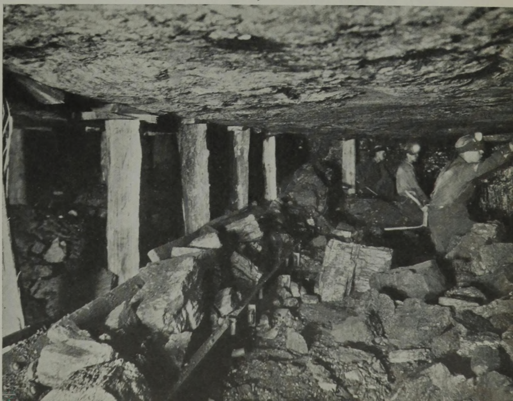
Loading Onto the Face Conveyor, Jewell Ridge.
