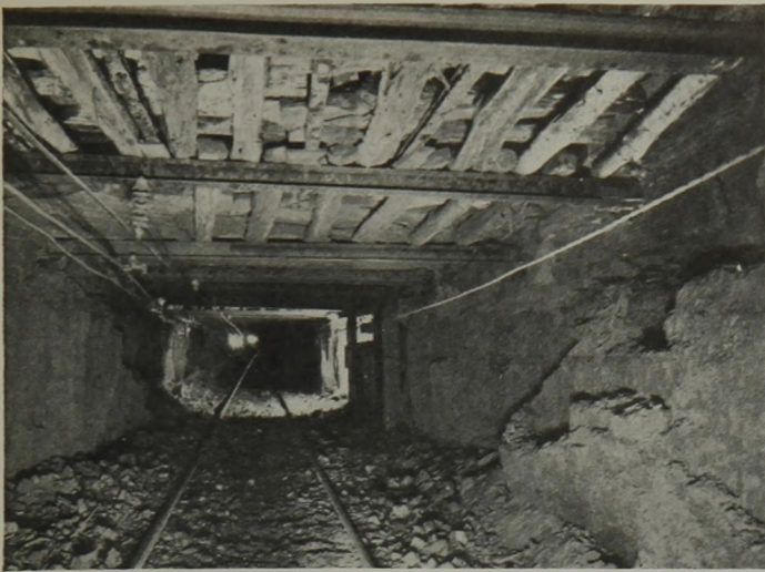
Fig. 6—Entry Timbering at Binkley No. 8, Showing Use of Individual Crossbars.
