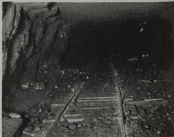
Left—Ties in This Main-Line Turnout Are 5½ Years Old. Right—New Treated Room Ties Generally Are First Laid in Switches Which Are Equipped With Throws. Before Being Discarded, These Ties Will Have Been Used From Three to Six Times Each.
