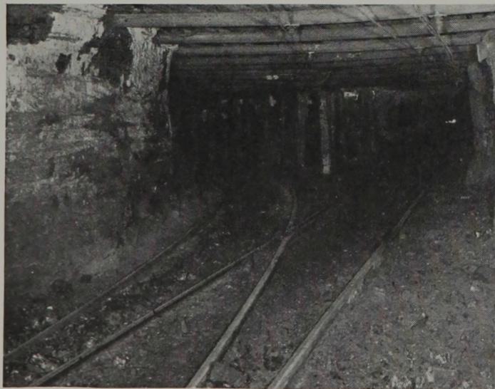
Left—Ties in This Main-Line Turnout Are 5½ Years Old. Right—New Treated Room Ties Generally Are First Laid in Switches Which Are Equipped With Throws. Before Being Discarded, These Ties Will Have Been Used From Three to Six Times Each.
