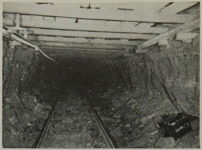
Fig. 7—Pin-and-Stringer Timbering at Dresser Mine, Walter Bledsoe & Co.
