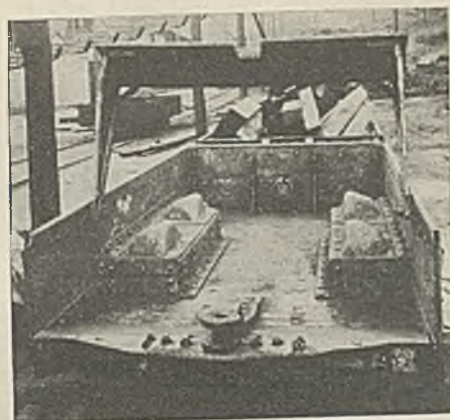
Use of an inside lifting endgate allowed making the car 1½ in. wider on the inside
