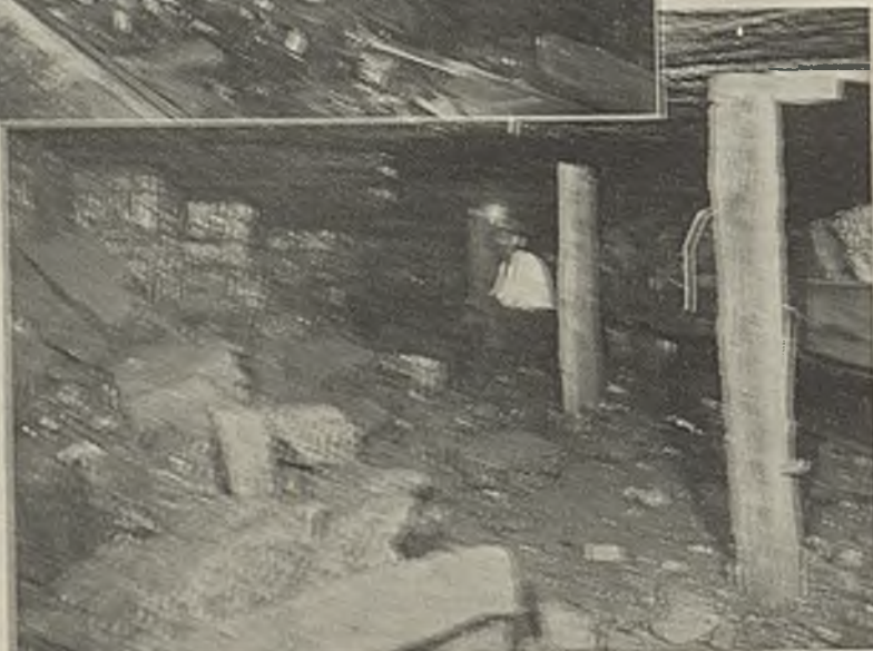
Mining a block at Bergoo No. 2 after a topcutting machine
