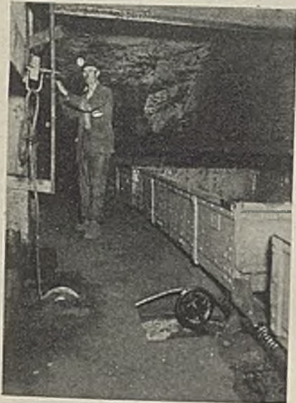
Couples a car and then pulls the lever to drop the trip one car length
