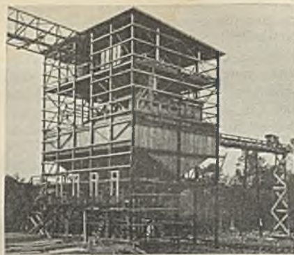
Fig. 2—Breaker, Gunton Coal Co., Bernice Pa., under construction
