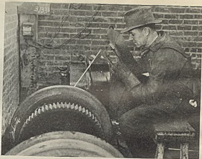
Using \frac{1}{4} -in. electrodes for welding filler bands into tires at the central shop of the Pocahontas Fuel Co.
