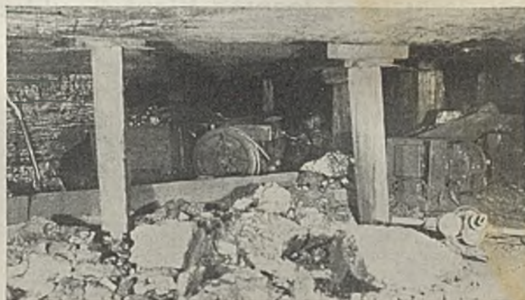
Face equipment as it appears from camera position A, Fig. 2
