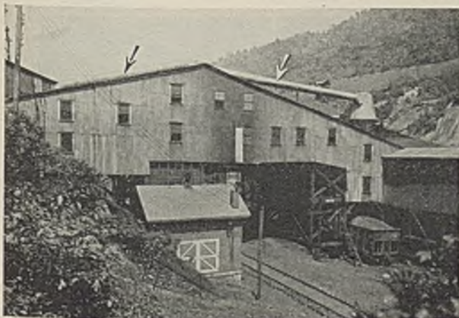
From a blower inside of the tipple and close to the slope opening a pipe carries the dust overhead to a cyclone collector
