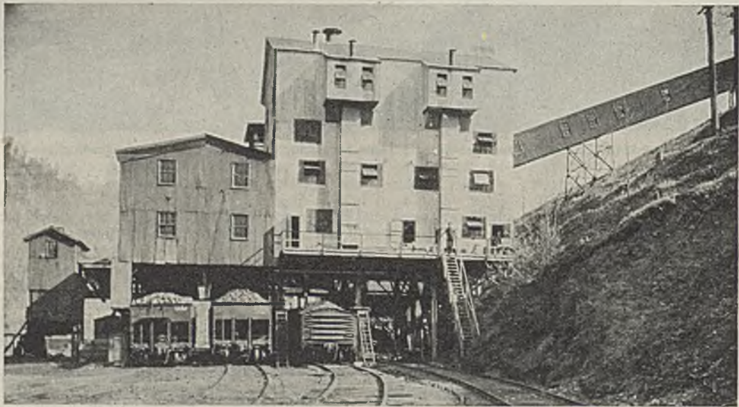
Lundale preparation plant with cleaning-plant addition in the right foreground. Retarding conveyor on right delivers coal from Lundale mine; coal from Big Vein mine comes across the valley by aerial tramway.
