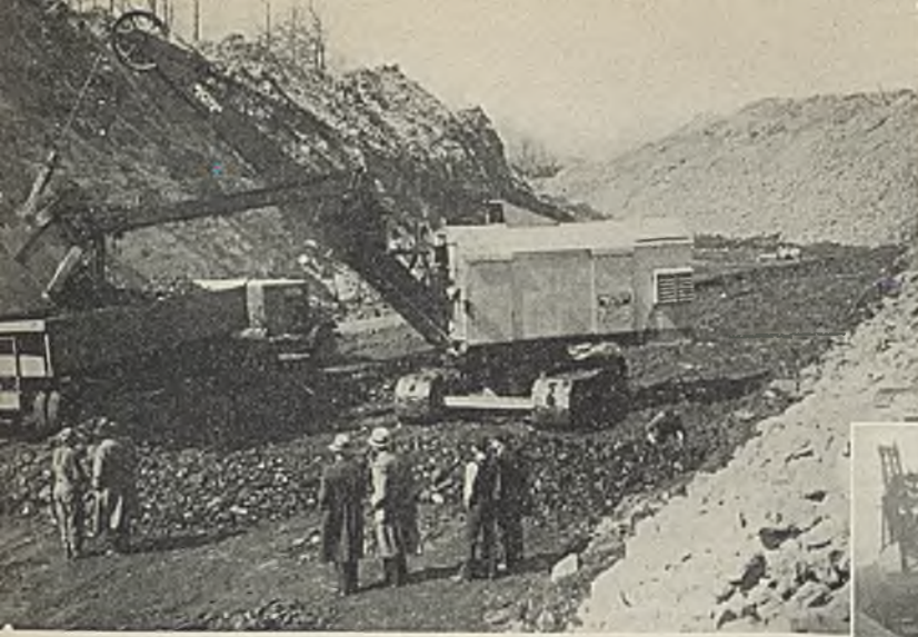
Coal is loaded by electric shovel with 5-cu.yd. coal-loading dipper into 25-ton tractor-trailer units
