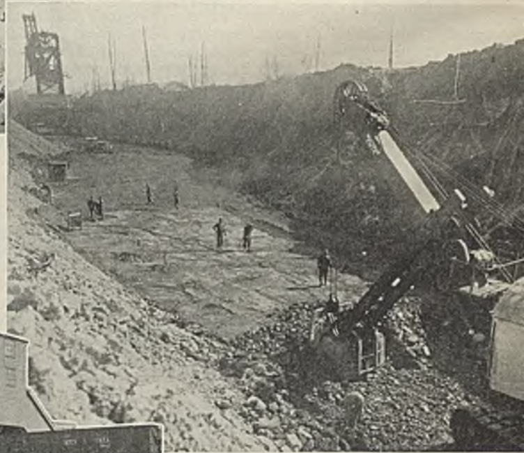
General view of pit, showing stripping; cleaning with bulldozer, hand shovels and compressed air; drilling and shooting; and loading
