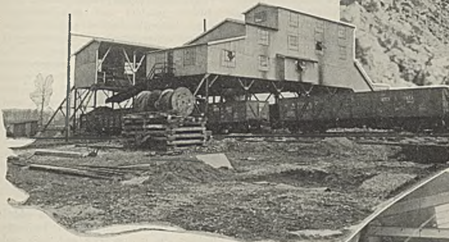
Bobolink preparation plant—main tipple at right, mixing conveyor and housing to the left
