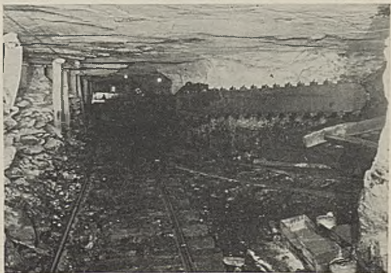
Track-mounted cutter entering a room at Mobley
