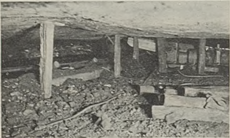
Room conveyor discharging onto main belt
