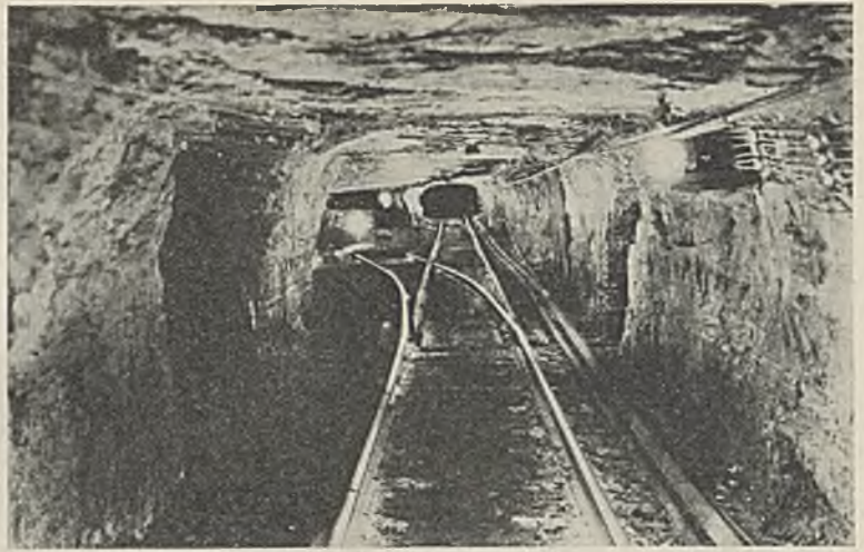
Main-line junction, Alexander mine. Track is laid with 75-lb. steel and cross rails. An electric switchthrower is installed (right) to operate the switch
