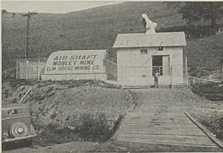
Fan installation and substation after removal to new Mobley air shaft near center of workings
