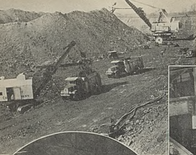
General view of No. 2 pit, showing stripping, loading and other activities
