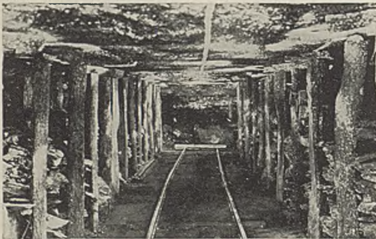
Safety in working places is assured by systematic timbering, car stops at the end of the room track and careful operation
