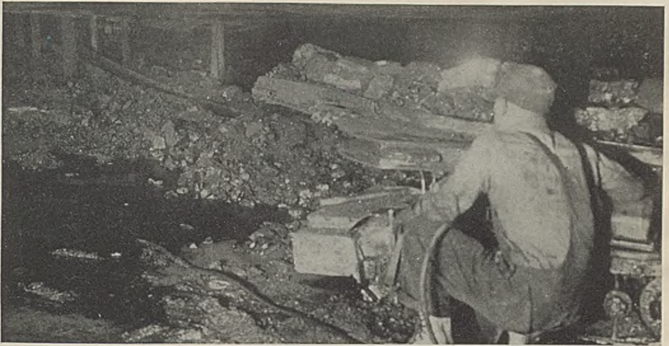
Loading machines at Goose Creek discharge into chain-and-flight conveyors which carry the coal to the main belt line extending to the tippie on the surface
