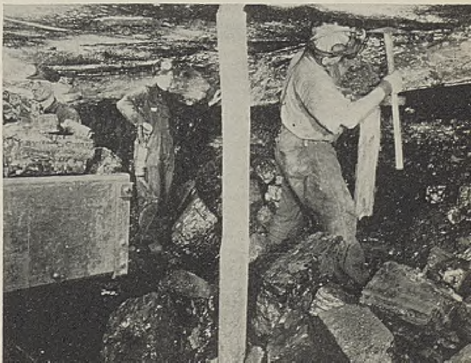
Safety at the face is assured by care in timbering and blocking the coal and the use of car stops, safety headgear and shoes, and goggles
