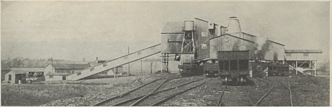
Sunlight preparation plant from the empty side
