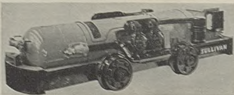
Sullivan Model 120 "Mine-Air" compressor
