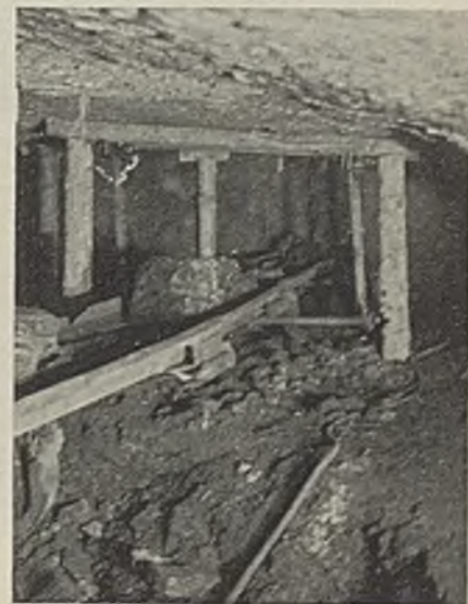
Hold-down installed on a conveyor at Peerless No. 3 mine
