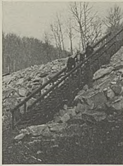
Even these steps of heavy treated timber reflect the engineering and thoroughness characteristic of the whole job
