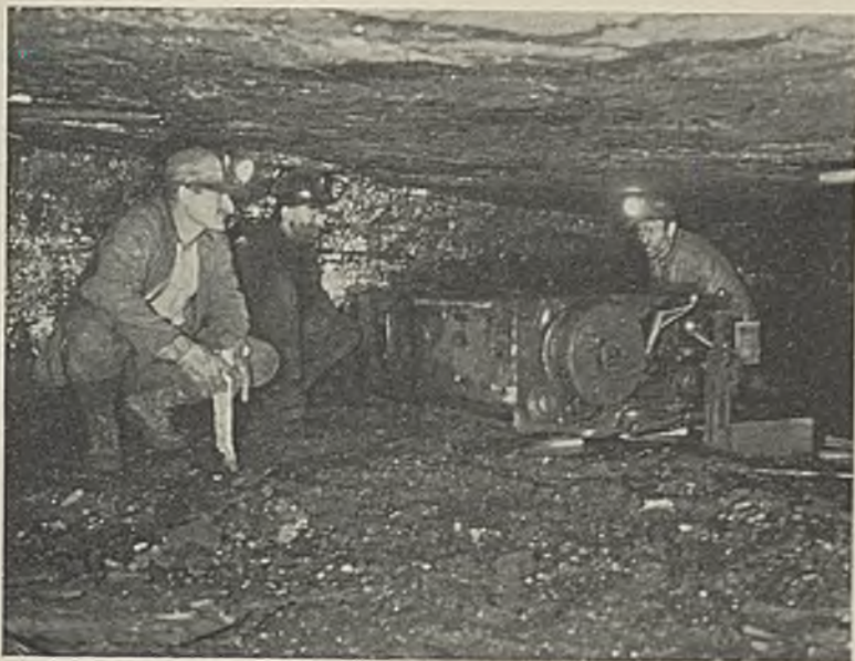
The foreman drops in to inspect the cutting, which is done with a low-vein machine
