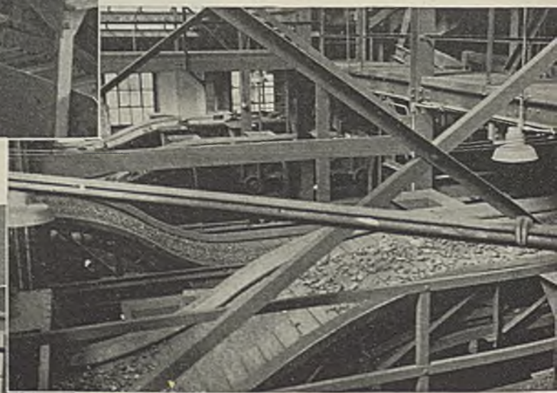
The four retractile-type picking designated, from near to far: nut, p and lump
