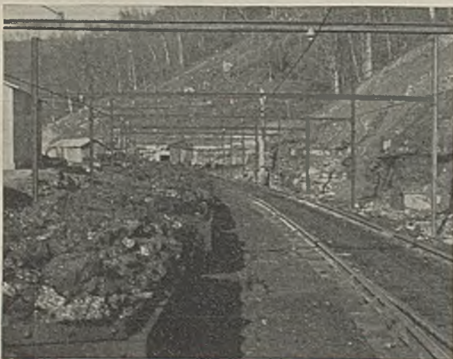
Mine-yard trolley wires are supported by posts of 40-lb. rail and crossbars of 30-lb. rail
