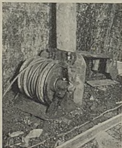
Retarder in place ready for service
