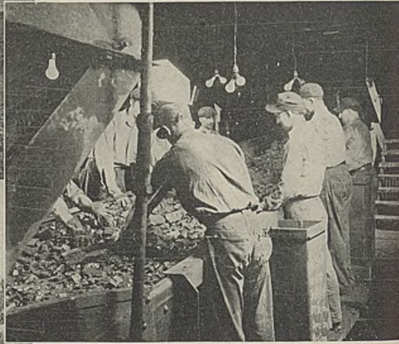
First stage in cleaning at Robinson Run: primary picking table in mine tippie.
