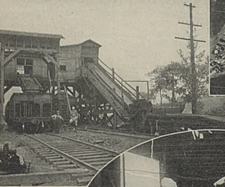
At the rail tippie, the coal is rescreened and given a final cleaning before going to the railroad cars.
