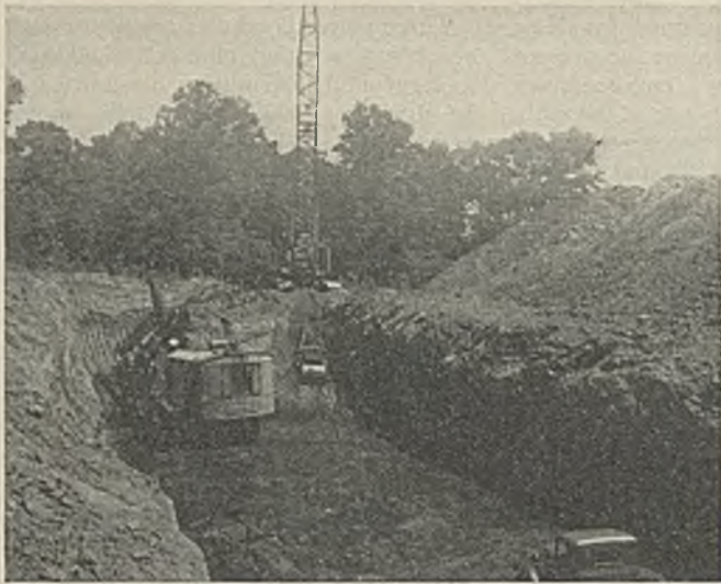
Left—Dragline making a box cut, with the shovel helping out in digging the soft overburden. Right—An example of the Sternberg tree-planting program. Trees on the spoil bank in the background are slightly more than one year old. Slips have been set out on the new spoil bank in the foreground, but are not yet large enough to show in the picture
