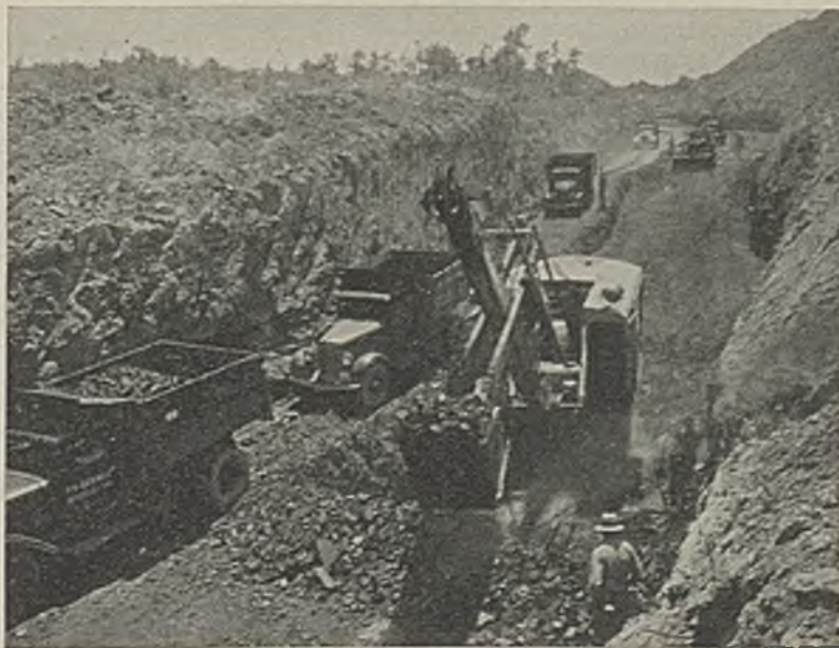
Loading shovel completing work in a box cut. Trucks move by the shovel on a 12-ft. berm of coal. The Angledozer used in cleaning off the coal appears in the rear
