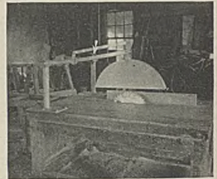
Saw guard in raised position (arrow points to locking screw)
