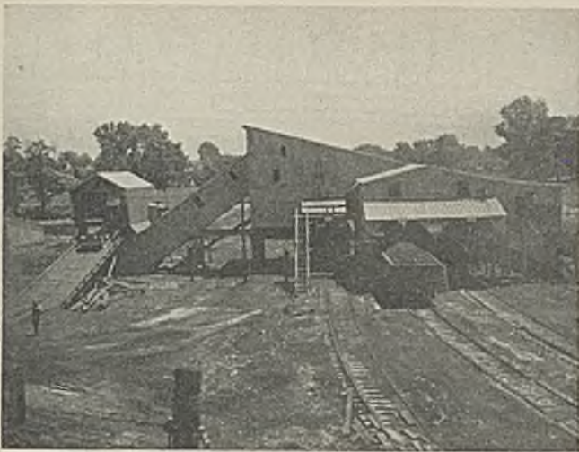
Sternberg preparation plant in the outskirts of Boonville. Trucks dump into the 25-ton hopper at the left
