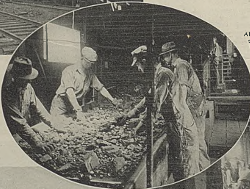
First stage in cleaning at Robinson Run: primary picking table in mine tippie.
