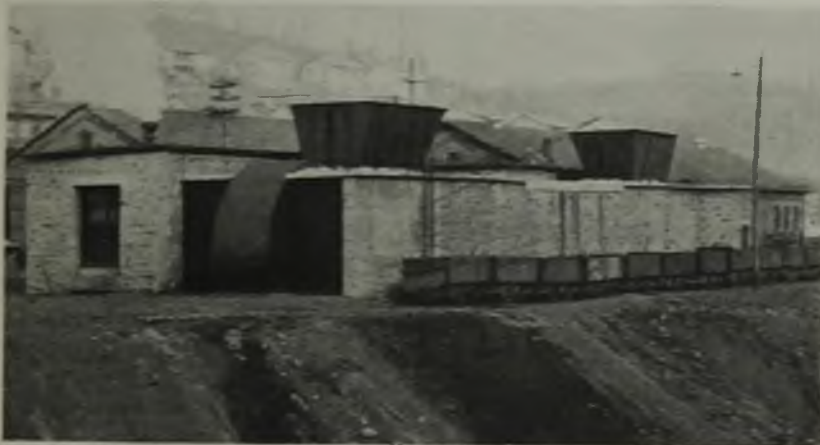
Fig. 3—Modern Double Installation of Primarily Exhaust Reversible Fans. One Fan Is Directly Connected to an Engine, and the Other Is Arranged for Belt Drive From an Electric Motor.
