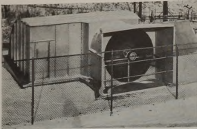
Fig. 1 (Left)—Now Using Only One Wheel, This Two Stage Aerovane Fan Installation of the Elm Grove Mining Co., Near Wheeling, W. Va., Is Operating as a Single-Stage Unit Delivering 77,000 C.F.M. at a 1.55-In. Water Gage and Consuming 28 Hp. This Fan Is Connected to a New 240-Ft. Deep Air Shaft at the Working Faces. Fig. 2 (Right)—Low-Cost Modern Fan Installation at Muskingum Coal Co. Mine, Near Zanesville, Ohio.
