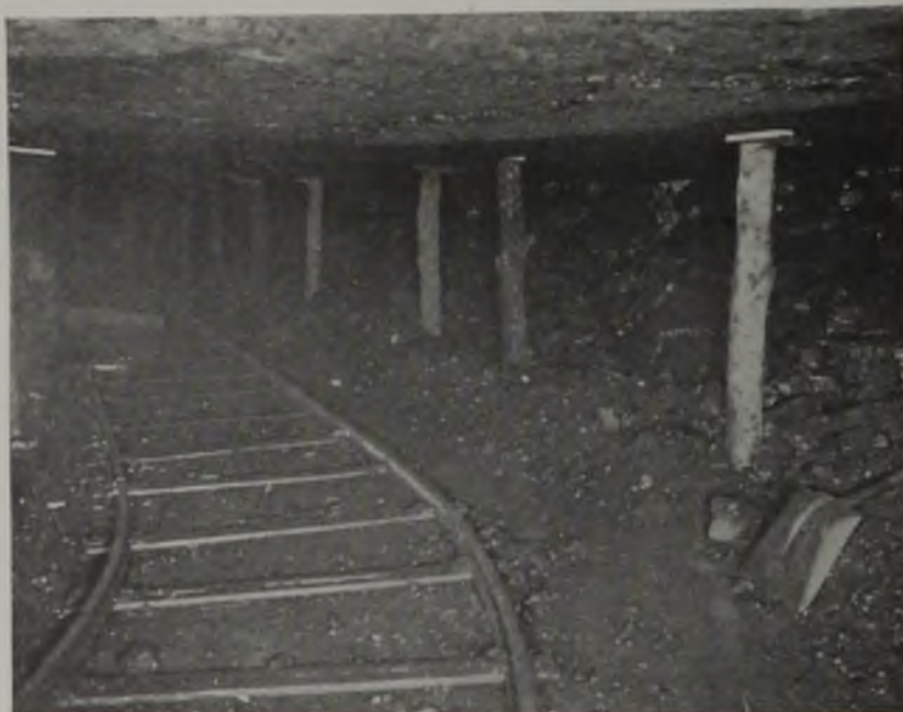
90-Ft. Place Ready for Loading.
