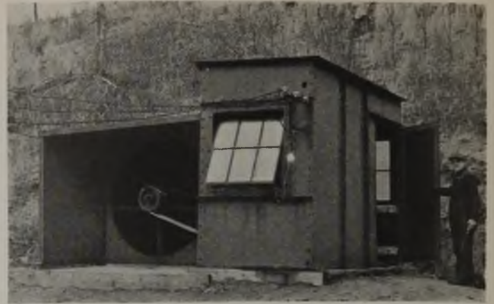
Fig. 1 (Left)—Now Using Only One Wheel, This Two Stage Aerovane Fan Installation of the Elm Grove Mining Co., Near Wheeling, W. Va., Is Operating as a Single-Stage Unit Delivering 77,000 C.F.M. at a 1.55-In. Water Gage and Consuming 28 Hp. This Fan Is Connected to a New 240-Ft. Deep Air Shaft at the Working Faces. Fig. 2 (Right)—Low-Cost Modern Fan Installation at Muskingum Coal Co. Mine, Near Zanesville, Ohio.
