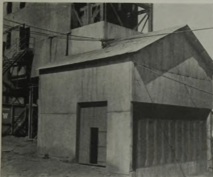
Radiator Building of Large Dimensions Provides Ample Room for Handling Materials in Case of Changing Skips or General Repairing.
