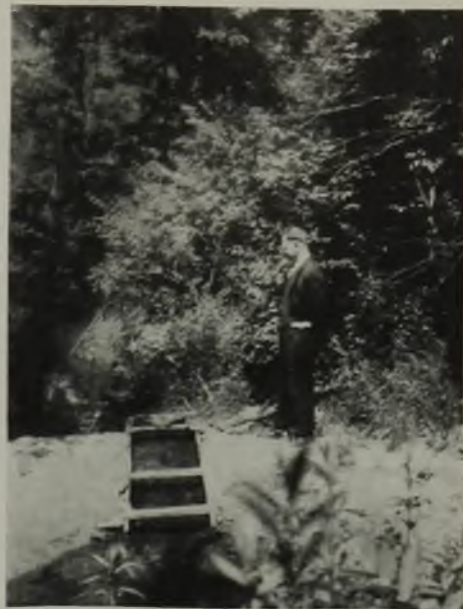
Earth Dam and Weir Box Seal by Raising Water Level.
