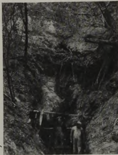
Preparations as Laborious as Sealing.
