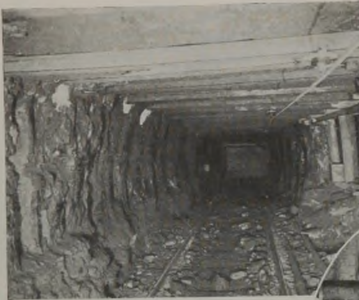
Main Entries Are Timbered With Steel Rails Using a Hitch Drill. Bottom Is Lifted for Height.
