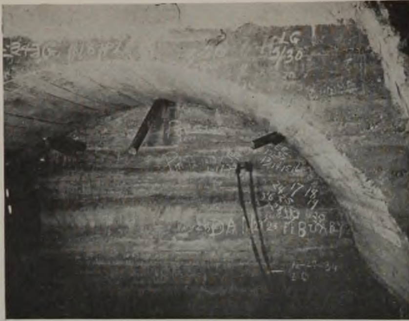
Completed High-Pressure Seal, Showing Pipes Used in the Blowing Operation
