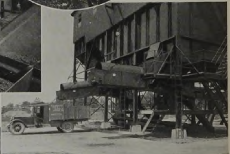
Close-Up of Truck-Loading Bins and Booms. Two Additional Booms and a Screenings Chute on Opposite Side Give Five Loading Points.
