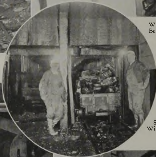
Main Entries Are Timbered With Steel Rails Using a Hitch Drill. Bottom Is Lifted for Height.
