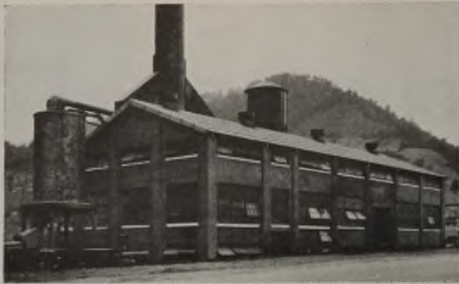
Steam Transports the Ash to the Round Dust-proof Bin, Which Is Vented to the Stack
