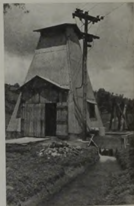
Lowest Impeller Is 304 Ft. Below Ground Level at the Pumphouse.
