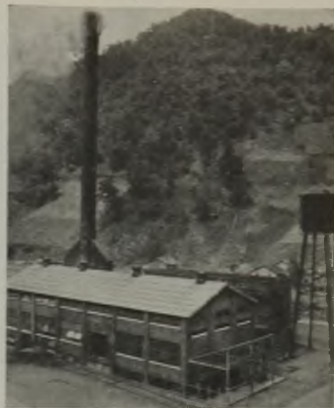
Outside Breechings Permit Simple, Continuous Hip-Roof Design. Between the Building and the Cooling Tower Back of It Are the Concrete Water-Storage Basins.
