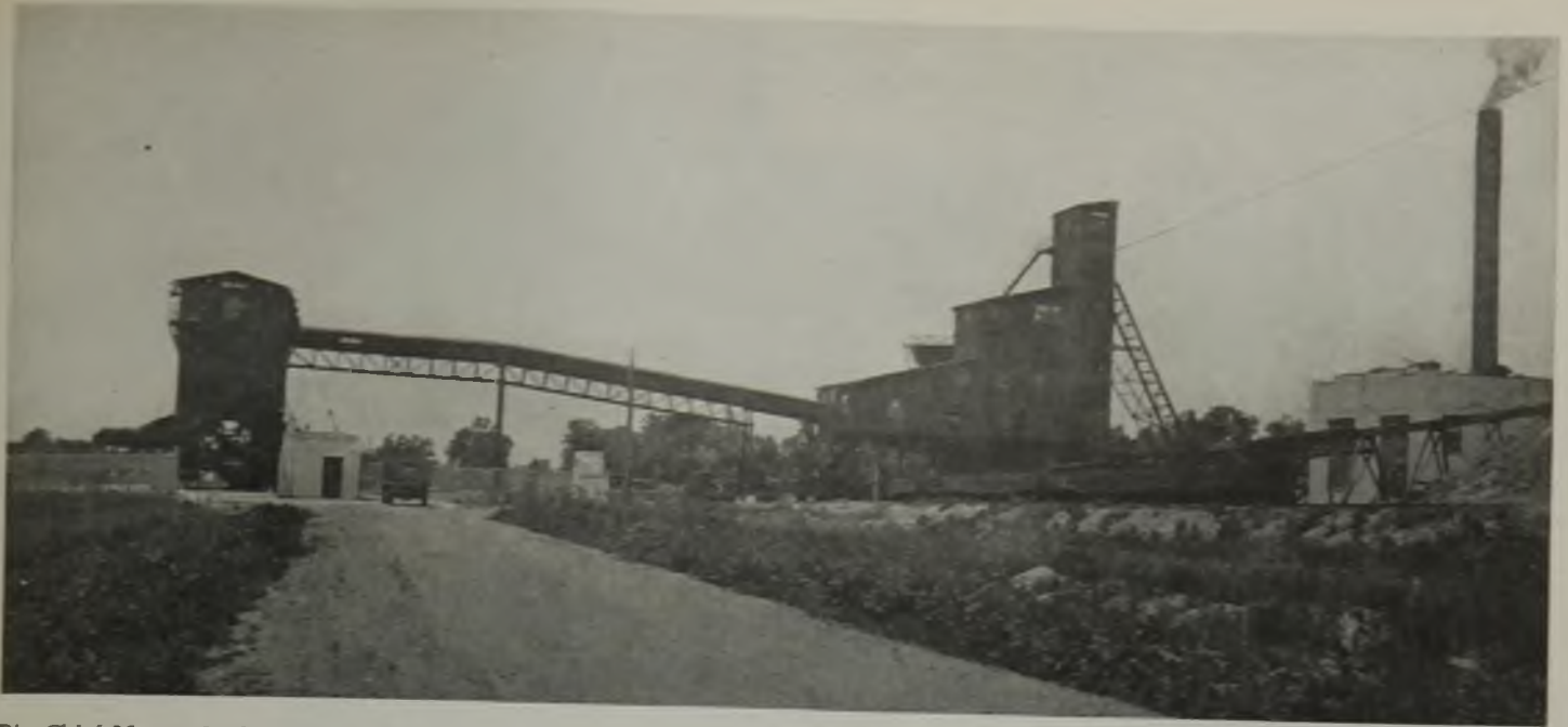
Big Chief No. 10 Surface Plant. Truck-Loading Plant and Scale House Are at the Left, Tipple and Washery in Center and Power Plant at Right. Mine Offices and Shops (Not Shown) Are Behind the Power Plant.
