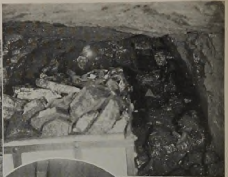
Working Face in Heading Being Driven in the Solid.
