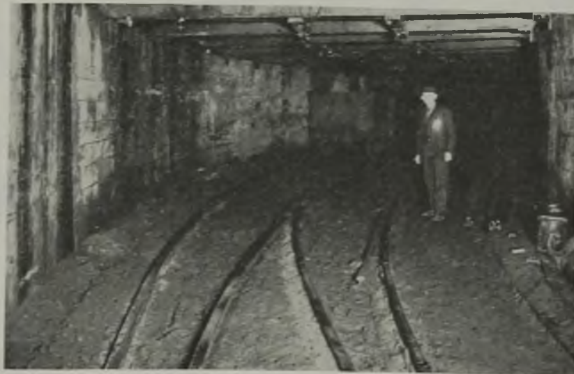
Fig. 1—Track Construction at Lehigh Navigation collieries is based on the use of 60-lb. rail and wood ties
