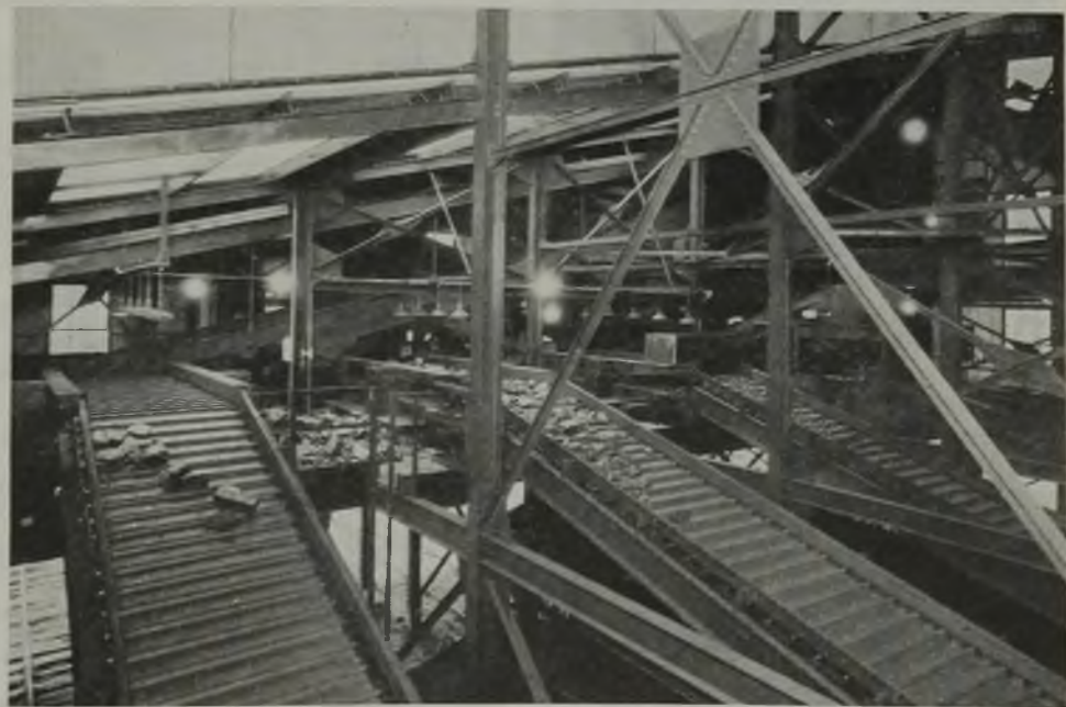
Special lighting is installed above the picking tables
