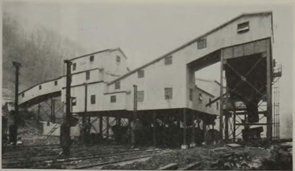
Looking down the track at the new plant. Car retarders and masts appear at left and the 100-ton rock bin at right
