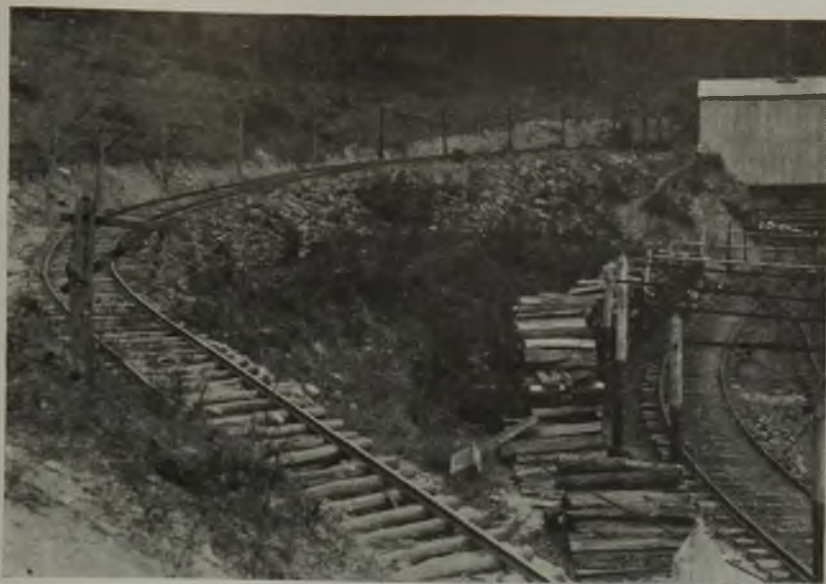
Up a steep grade the spur track at the left leads to the sand-house floor level
