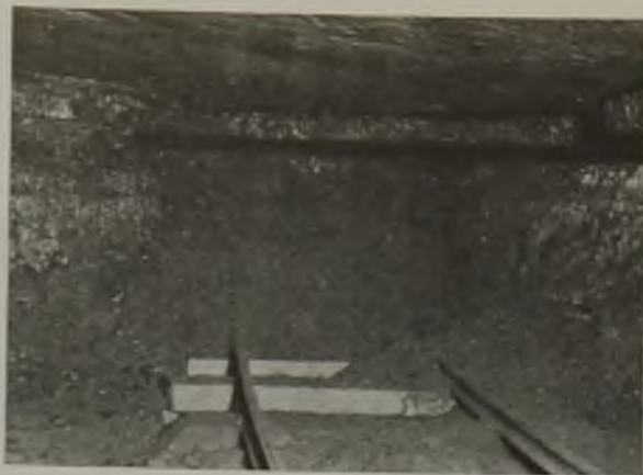
Left, cutting out the parting has just been completed in this room; right, heading with cut completed in the parting; here the bottom rock and part of the bottom coal is taken to provide height for main haulage
