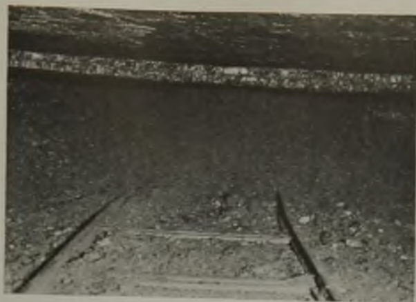
Left, cutting out the parting has just been completed in this room; right, heading with cut completed in the parting; here the bottom rock and part of the bottom coal is taken to provide height for main haulage
