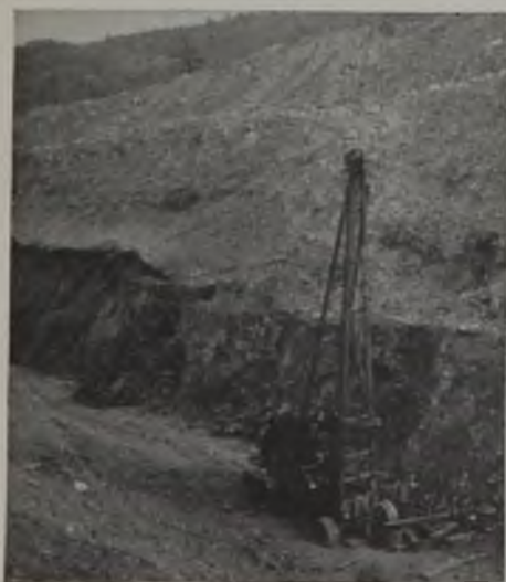
Fig. 6—Neyers north dip stripping, Nesquehoning, showing drilling for the final rock cut and also pillars of coal standing up against the bottom rock
