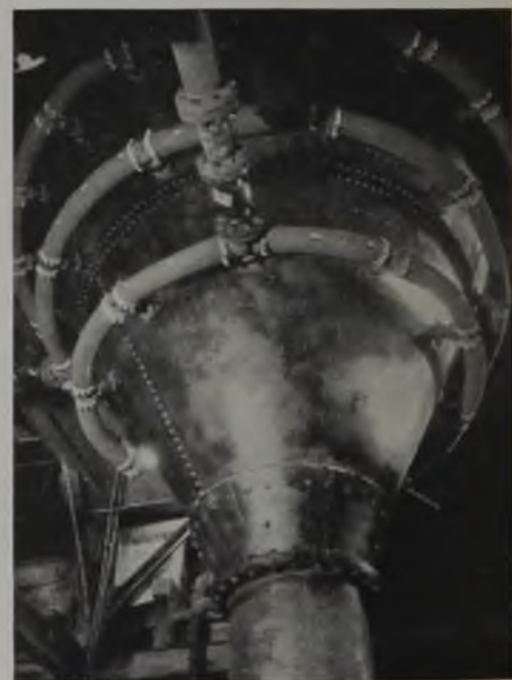
Three Lehigh Navigation breakers are equipped with cones for cleaning
