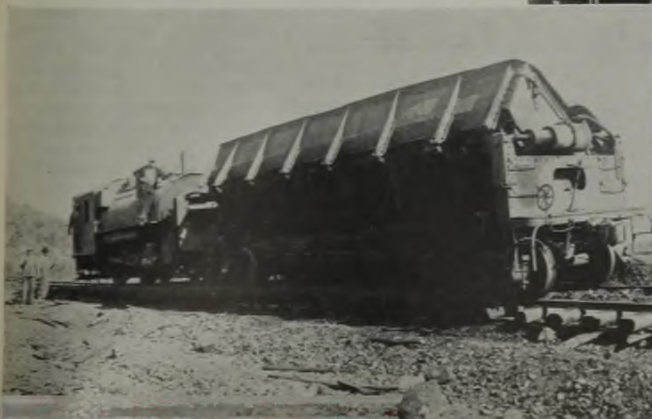
Side-dump cars hauled by steam locomotives are used for refuse disposal at Lehigh Navigation collieries
