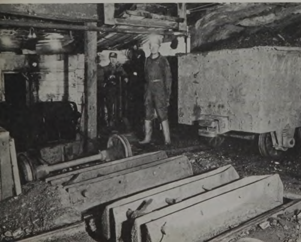
Transfer car handling loaded cars, No. 9 shaft, Coaldale colliery
