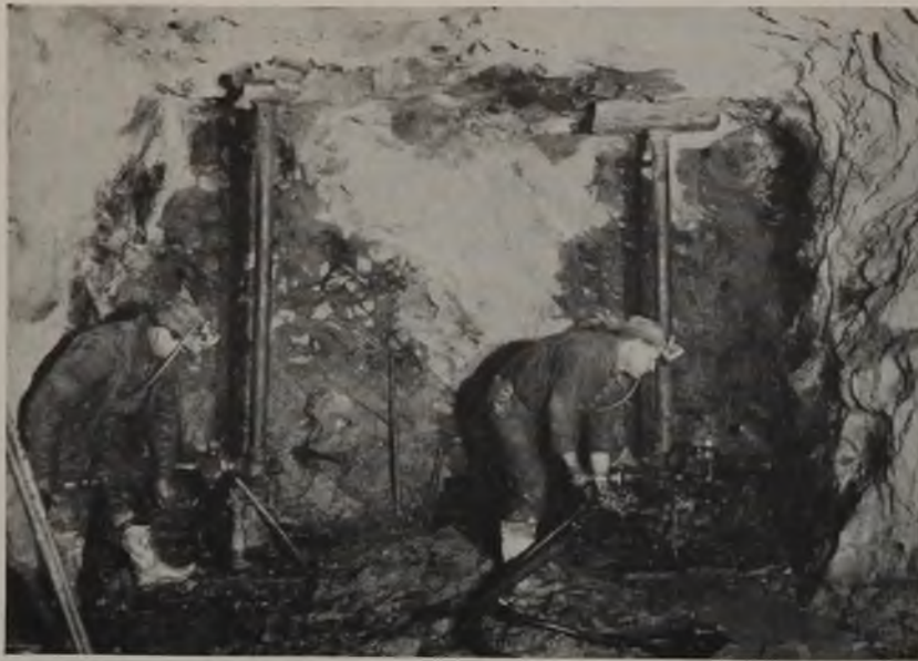
Contractor's men using water-leyner air drills in driving a tunnel on the fifth level, Lansford
