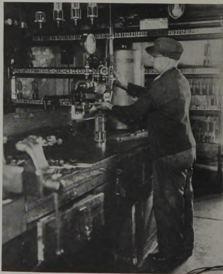
Fig. 2—A lamp is cleaned and filled in 75 seconds
