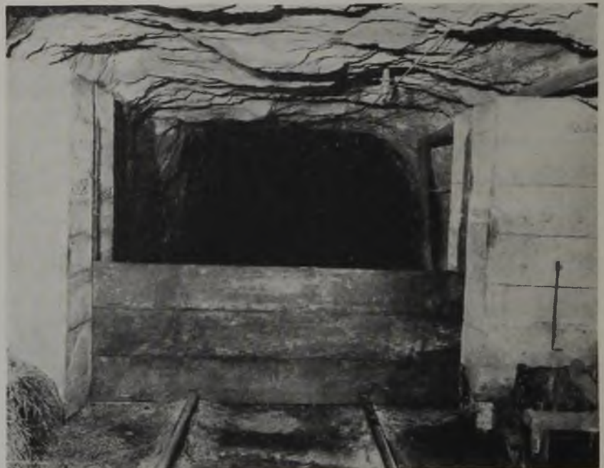
To demonstrate this concrete-and-plank dam in Lansford, No. 6 shaft, third level, several of the lower planks were taken from their storage place along the rib and dropped into the grooves in the concrete abutments
