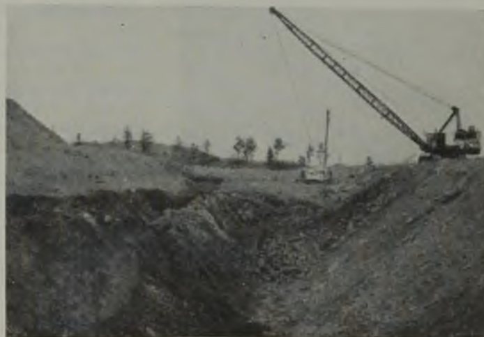
Fig. 3—Dragline making rock cut at Mammoth south dip strip-ping, Lansford colliery
