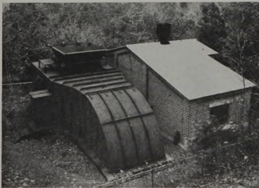
The motor room of this fan at No. 3 shaft, Nesquehoning, serves also as a d.c. substation. Both controls are full-automatic
