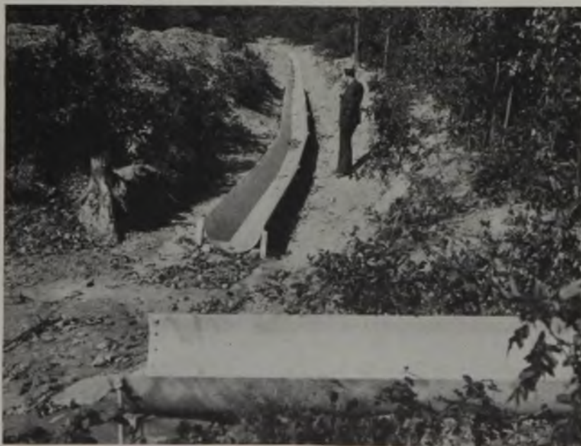
Half-round steel flumes such as these at Tamaqua conduct water over crop falls and surface cracks
