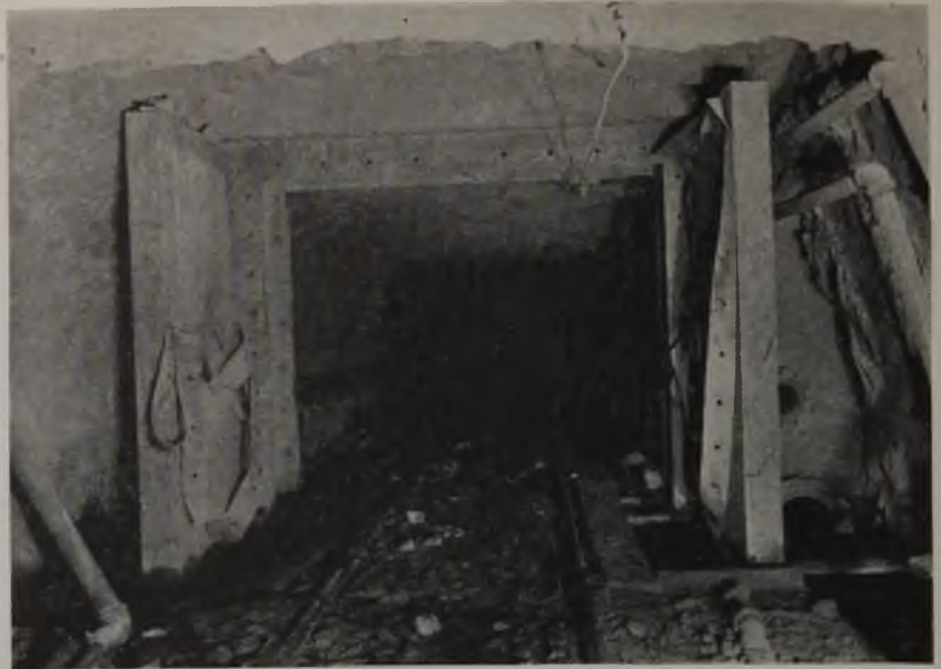
Rubber gaskets are hanging loosely in place on this side-hinged steel-door flood-control dam in Lansford colliery, No. 6 shaft, fifth level
