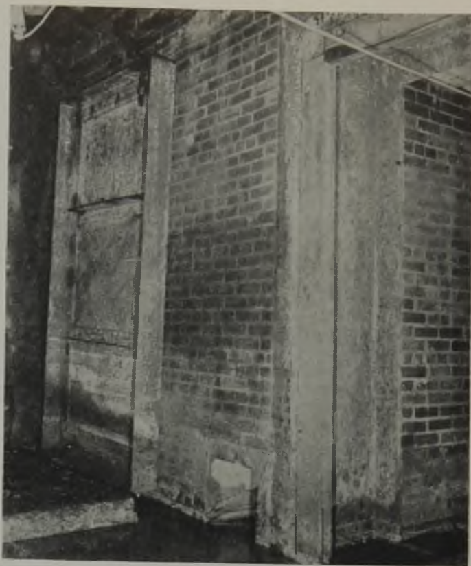
One side of the flood-control dam, No. 3 level, south side, Tamaqua. Each door half rolls on an overhead track into a recess in the rib
