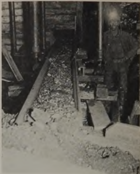
Shaker conveyor driving coal gangway at Alliance colliery
