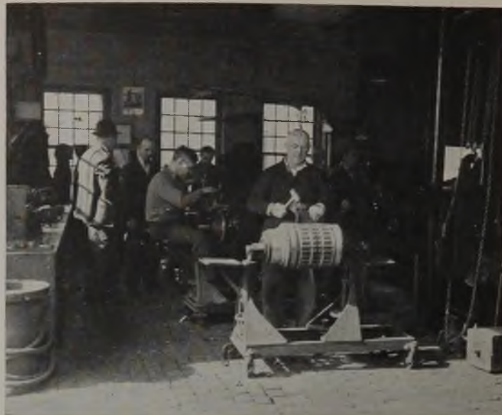
One hundred locomotive armatures were repaired in the electrical shop in 1934
