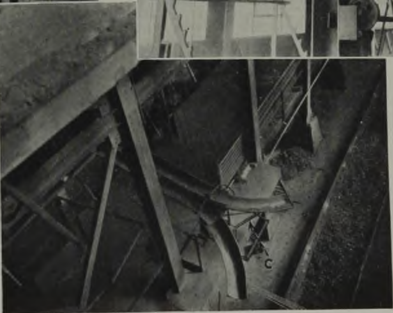
Fig. 7—Carriage run out and extensible spouts in position for loading
