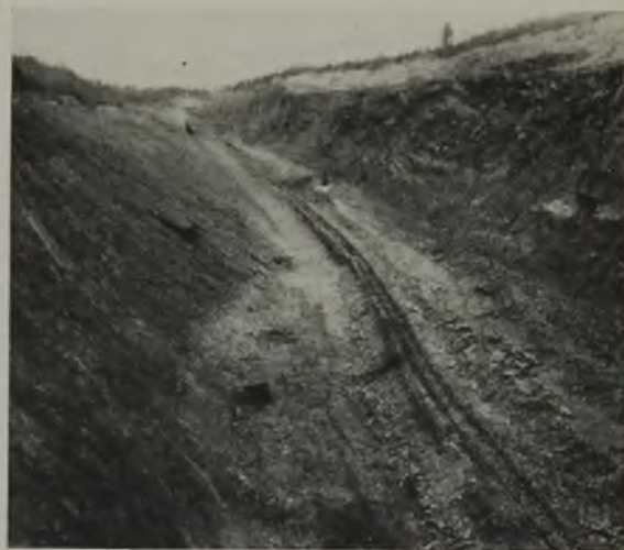
Fig. 1—Hell's Kitchen strip-ping, Nesquehoning colliery. Sixty feet of coal in the bottom is yet to be loaded
