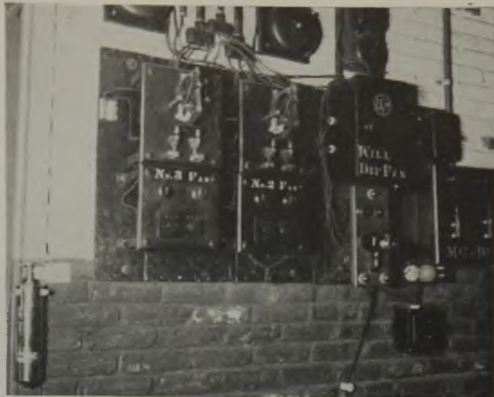
Control buttons, signal lamps and alarm bells for the three mine fans and for an outlying motor-generator are grouped in the main substation at Nesquehoning
