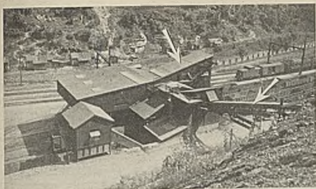
Arrows Point to Separator Addition and Shaker Trough Over Highway
