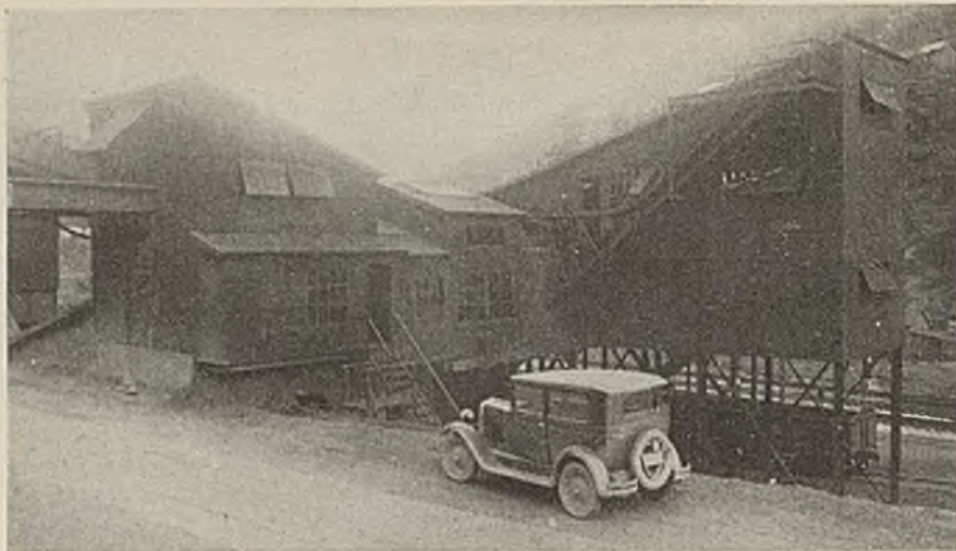
Showing Raw Coal and Refuse Conveyor Mounted on Outside Wall of Separator Addition
