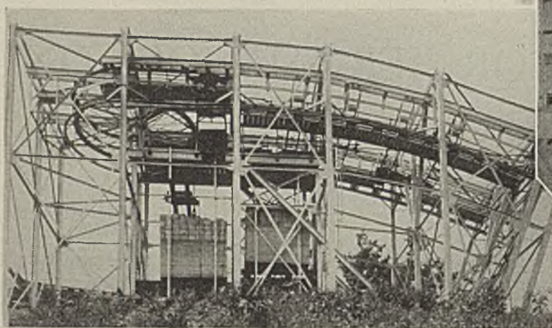
Tail Terminal Where Buckets Turn Around and Traction Ropes Are Anchored to Weights
