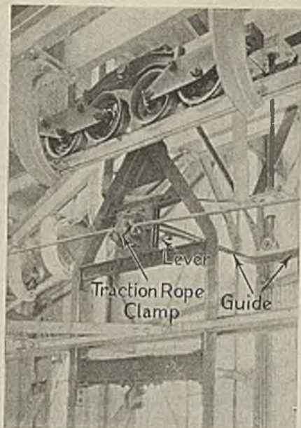
Bucket Suspension Frame Being Clamped to the Traction Rope
