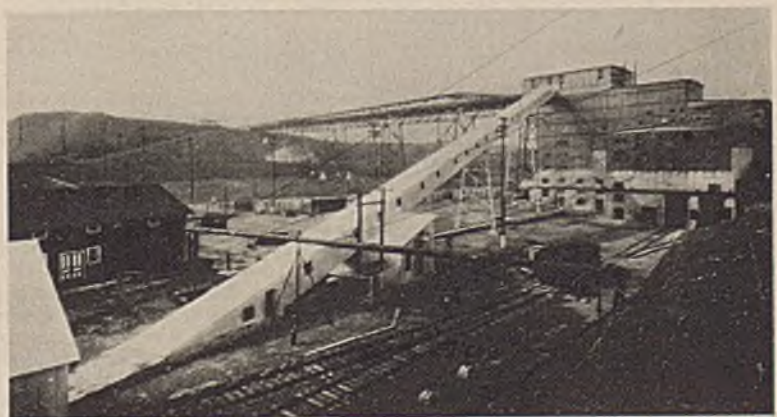
Pittston No. 9 Colliery, Showing the Contrast between Aluminum-Painted Surfaces and the Old Finish. When This Picture Was Taken, Only the Conveyor Gallery in the Foreground Had Been Painted.
