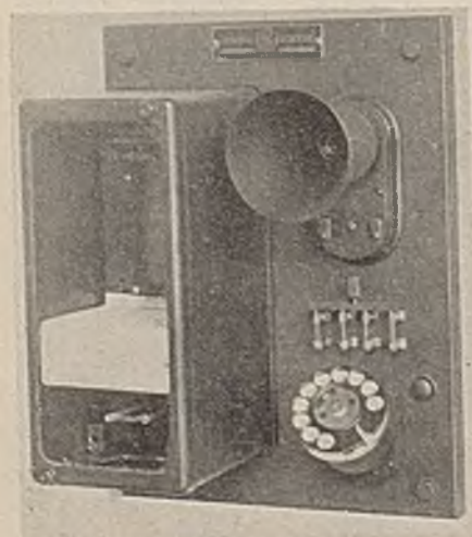
Dispatcher's Control Panel, Automatic Supervisory Equipment
