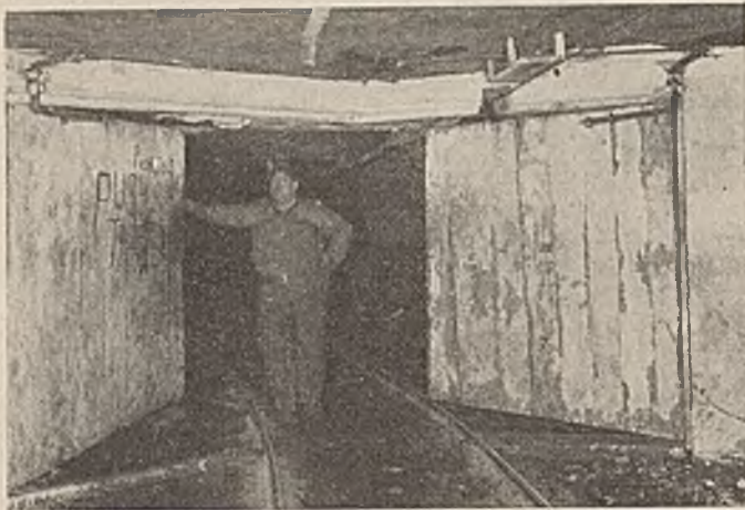
Opening One Side of the V-Door Automatically Opens the Other
