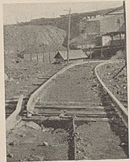
Fig. 2—Switch and Actuating Fulcrum
