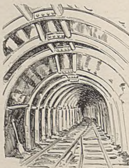
Fishplated Steel-Rib Arches With Struts Between
