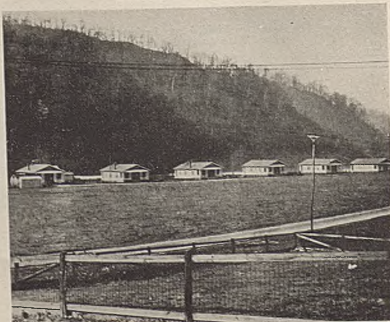
A Few of the Kentenia Houses
