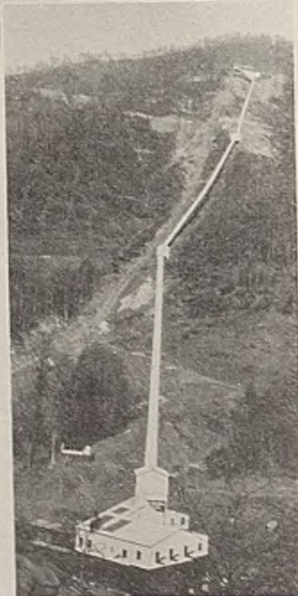
1,200 Ft. Difference in Elevation Between Mine Track and Railroad; Sky-lights in Tipple Roof Are Above Main Screen and Picking Tables
