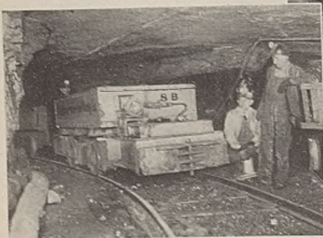
One of the Storage-Battery Locomotives in a Room Neck; Note the Wide Radius of This Track Turnout
