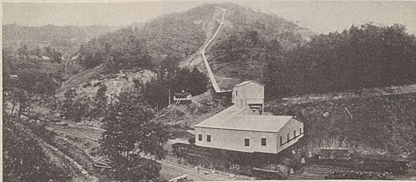
Panoramic View of the Mayflower Surface Plant; Conveyors Lower the Coal Nearly Three-Quarters of a Mile
