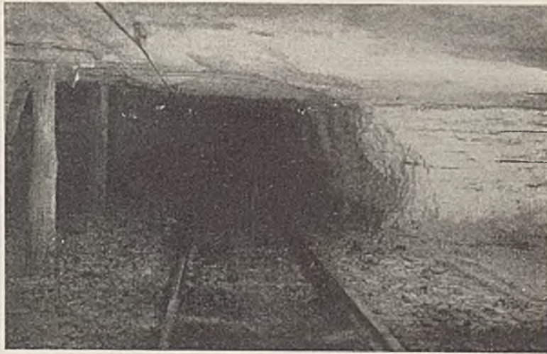
Light Is Projected Into Manhole but Shielded From View Along Track
