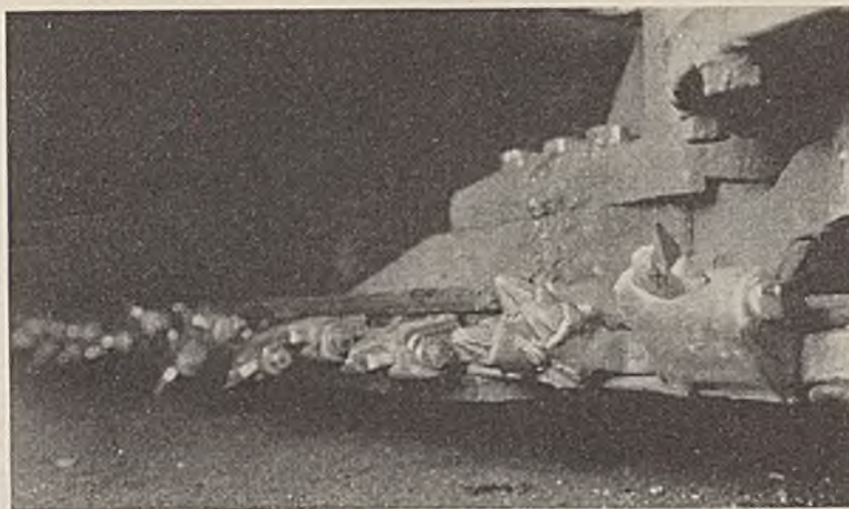
In Position for Undercutting. This Machine, of the Track-Mounted Type, Is Equipped With a Special Chain. Note the Core Breaker. Chain Was Under Test When Photograph Was Taken
