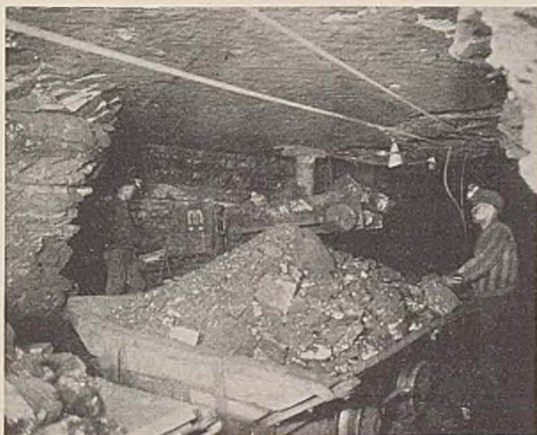
Fig. 3—Motor Crew Picking and Trimming Longwall Coal at Loading Conveyor
