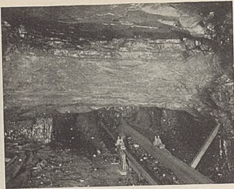
Fig. 5—Duckbill Loading in Haulage Heading of Longwall Entry
