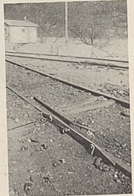
Treadle on Near Track Counts Coal Cars and One on Far Track Counts Slate
