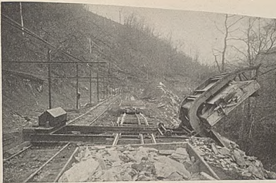
Car in Full Dumping Position
