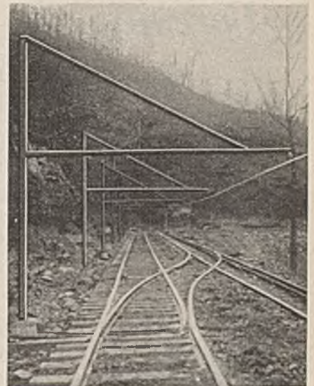
Permanent Supports in Unfilled Ground
