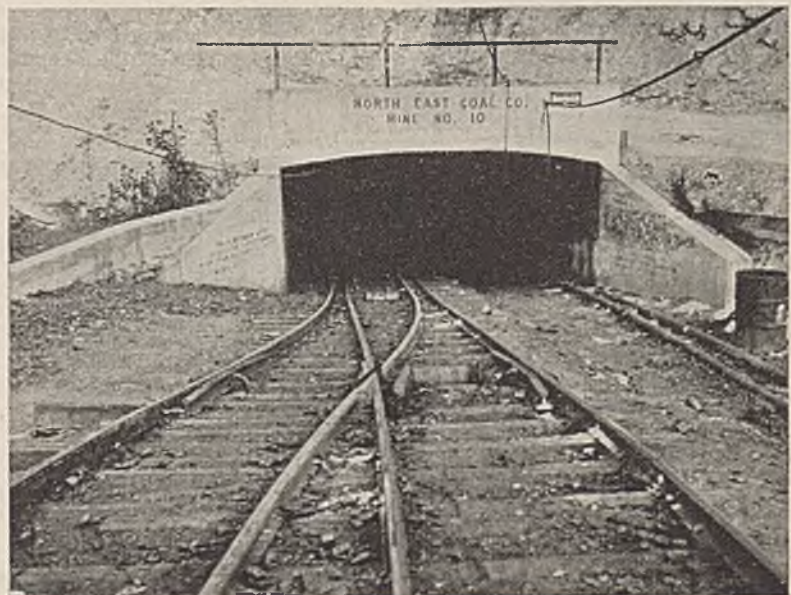
Empty Track Laps Over Onto the Loaded Track at the Portal
