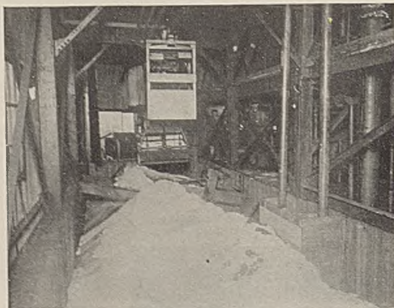
Fig. 4—Bin Alongside Washer Building, Equipped With Monorail Crane, Reduces Sand-Handling Labor to a Minimum
