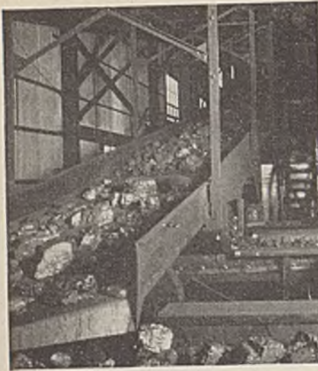
The Picking Tables Empty Directly Into the Retarding Conveyor
