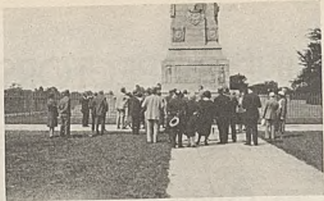
At the Base of the Monument at Jamestown
