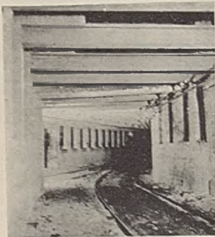
Fig. 1—Under Relatively Low Roof, H-Beams Are Placed on Pillasters
