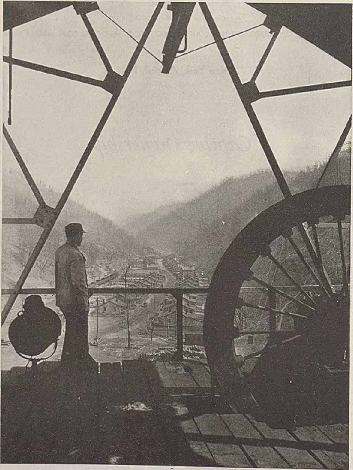
Dehue Headframe Looks Out Over Village in Valley
