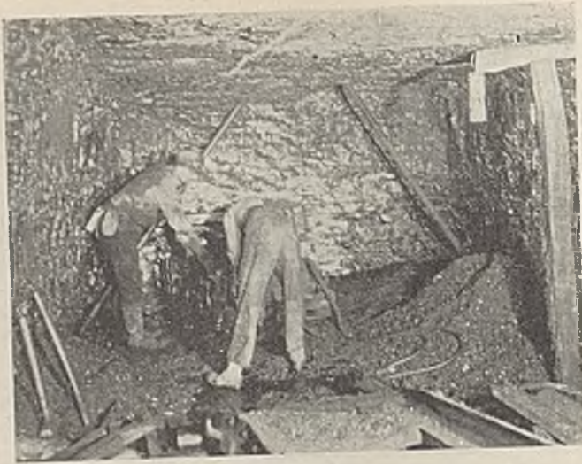
Shortwall Machines Are Used in Cutting Secondary Headings and in Robbing Pillars
