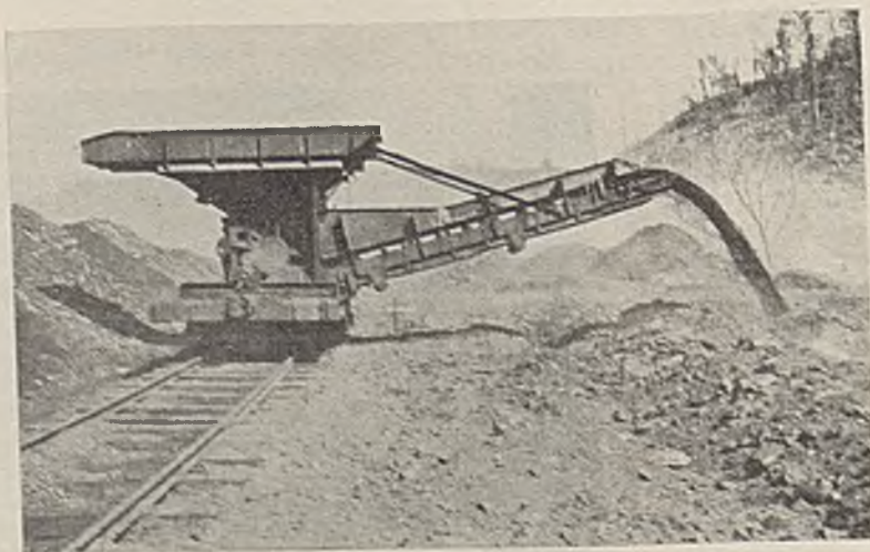
Fig. 6—Discharging Refuse on the Spoil Bank
