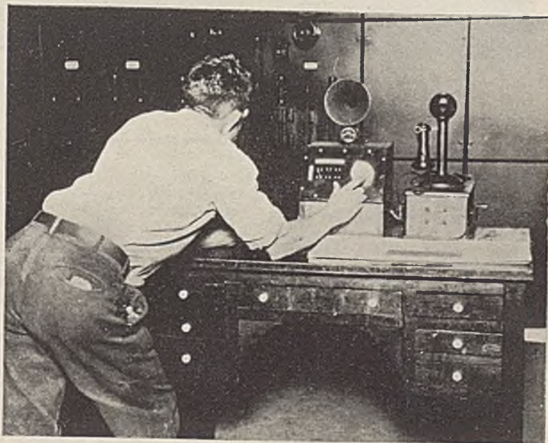
Fig. 1—Starting No. 2 Substation by Dialing a Code From No. 1
