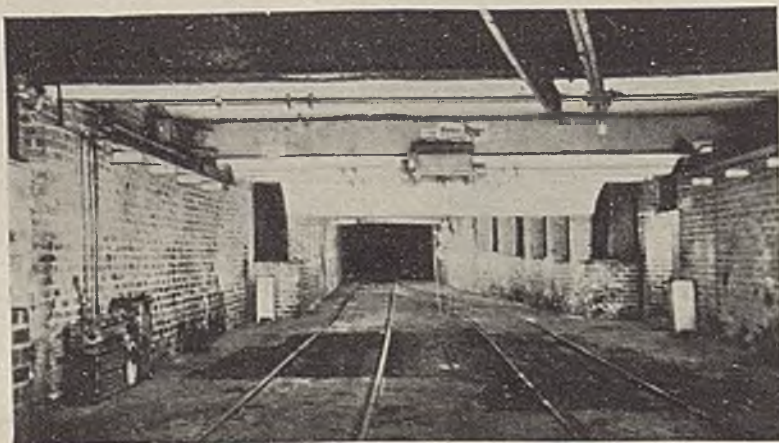
Underground Locomotive Barn Equipped With Two Track Pits and an Electric Crane
