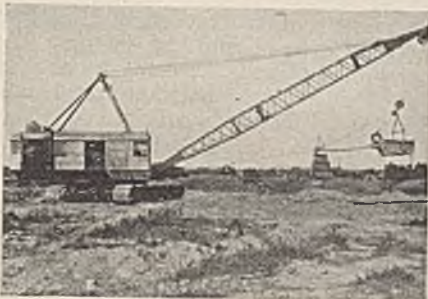
Class III, Diesel Dragline Excavator Equipment
