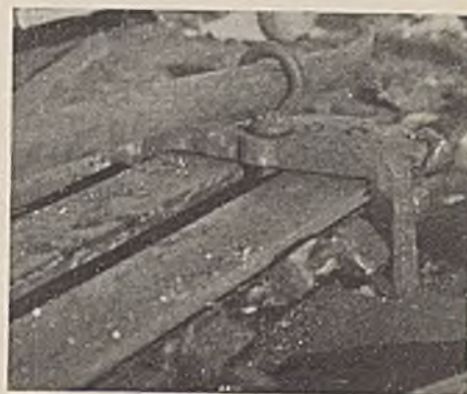
Fig. 1—Clamped, and Locked by Jack Pipe
