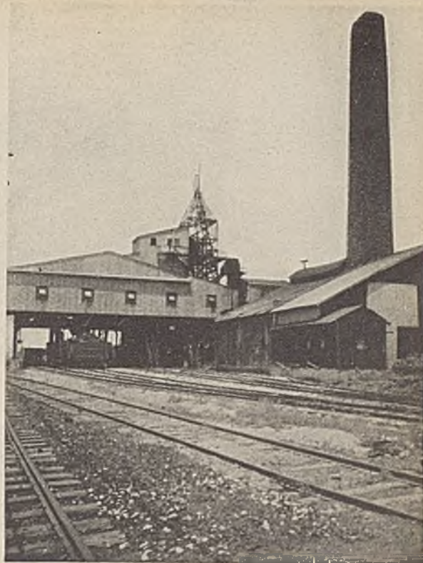
Tipple Was Modernized and Generating Equipment Added to Power Plant
