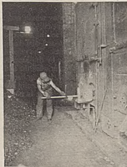
Firing Fuel for Mine Power
