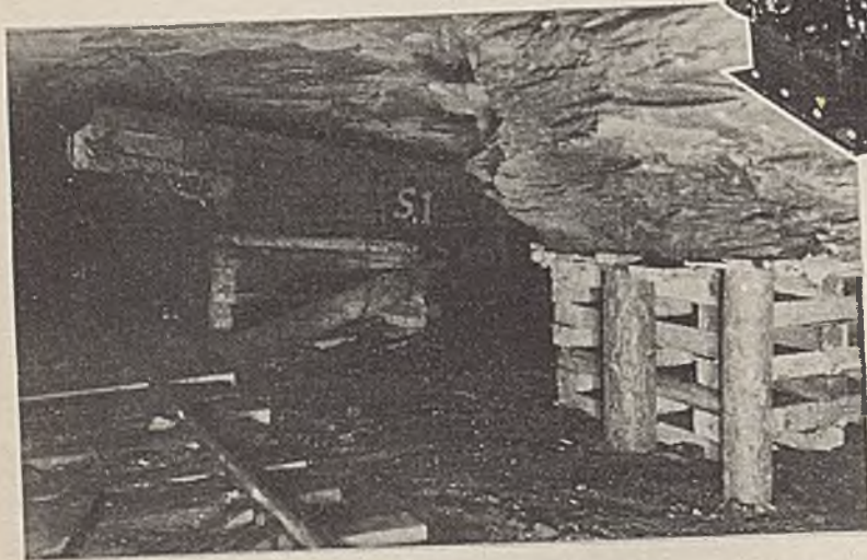
Fig. 3 — Head of Room Conveyor With Cribbing to Help Sustain Air-course Ribs
