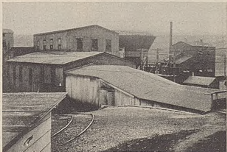
Close-up of Preparation Plant
