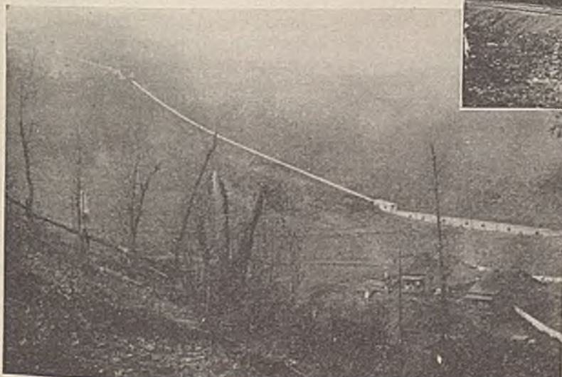
Fig. 5—The Three Sections of the New Conveyor System
