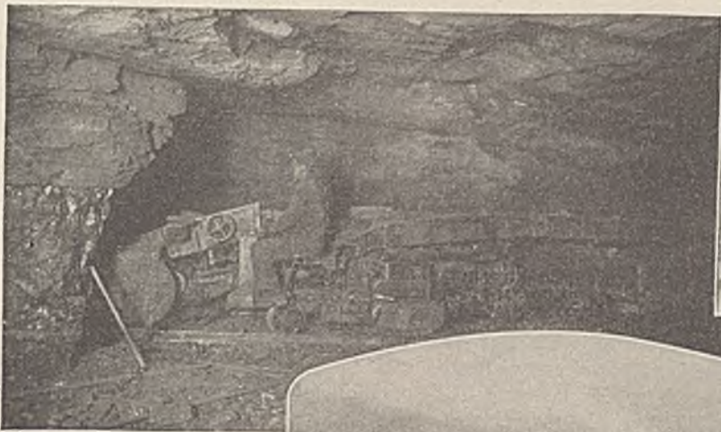
Fig. 2—Loading Rock in a Breakthrough
