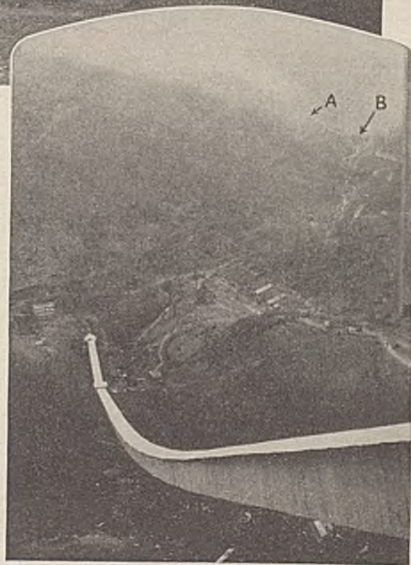
Fig. 4—"A" and "B" Are the Headhouse and Tipple, One Mile by Tramroad From the Bottom of the Conveyor
