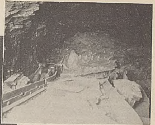
Fig. 3—Head of Machine Loading Rock Shot From Top in Breakthrough
