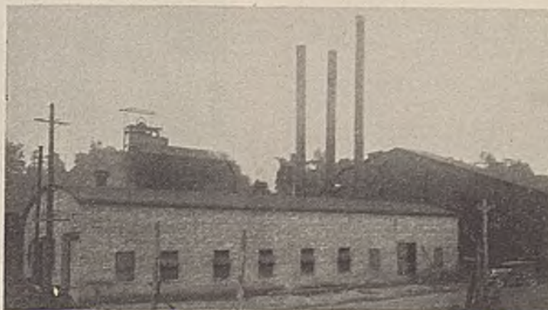
Power Plant Stands Close to Tipple, Fuel Being Delivered by Short Conveyor. Headframe in Center Background Belongs to Another Company
