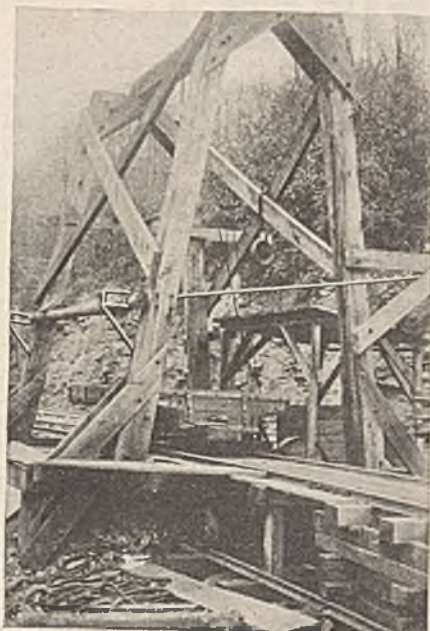
Fig. 2—Empty Car Back in Normal Position
