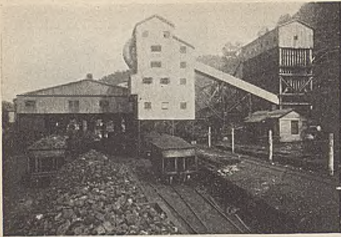
Tipple, Dry Cleaning Plant, and Storage Bin at No. 4 Mine
