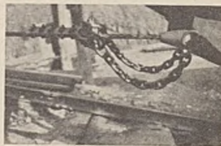
These Chains Are Too Loose
