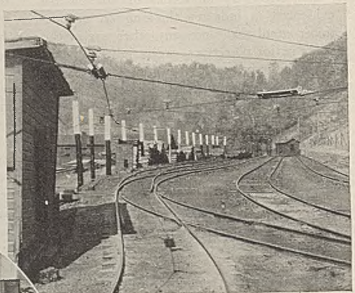
Fig. 3—Two-Point Control of One-Track Switch
