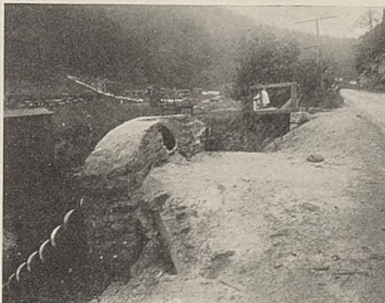
Sand Is Unloaded From Trucks on a Highway That Overlooks the Plant
