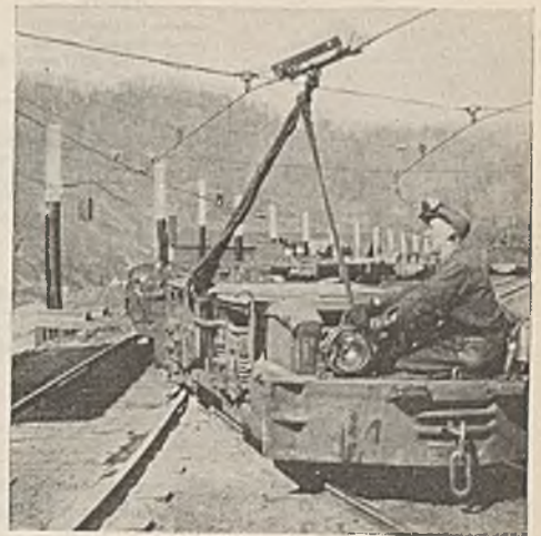
Fig. 6—Track Switches Are Operated by Manipulation of the Controller Handle
