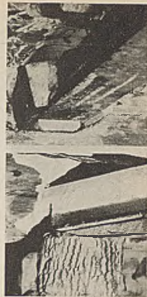
A Contrast in Timbering Methods—Above, the New, Safe Way; Below, the Old, Dangerous Way
