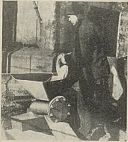
Pouring Sand Into the Hopper
