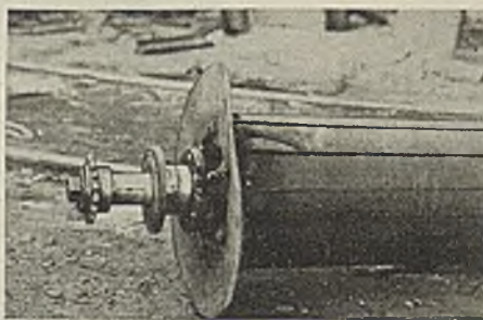
Fig. 8—Collector and End Rings in Good Condition After Four Years' Service
