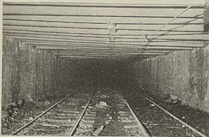
Above—Double-Tracked Entry Walled With Blocks
