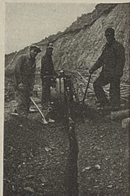
Where Kerf Is Cut Track Is Not Disturbed
