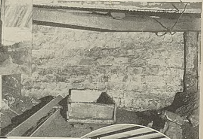
Below—Brattices Made From Blocks Improve Ventilation Efficiency
