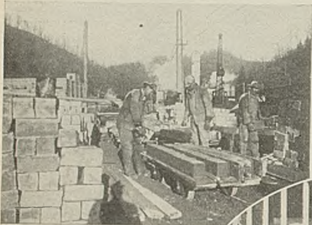
Above—Stripping Molds and Putting Day-Old Blocks in Stockpile
