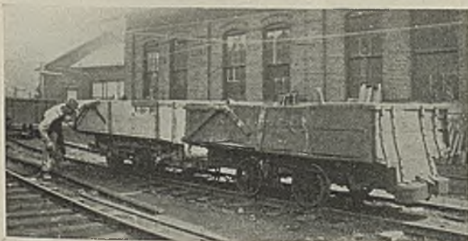
Same Irons but New Trucks; Car at Right Ready to Enter Shop and That At Left Just Out
