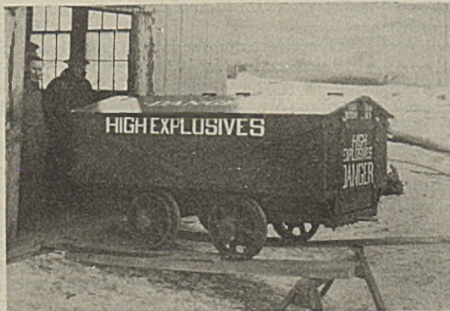
Car With Inner Insulated Box for Explosives
