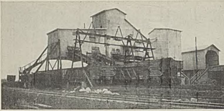
Old Glory No. 17 is served by a five-track all-welded steel tippie with three loading booms
