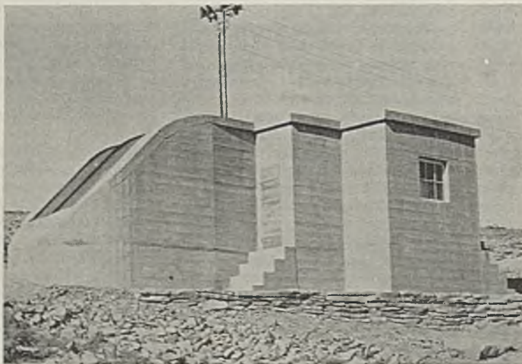
Concrete fan house at Winton, Wyo., Union Pacific Coal Co.
