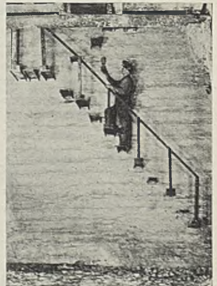
Climbing up to inspect high seal can be done in safety.
