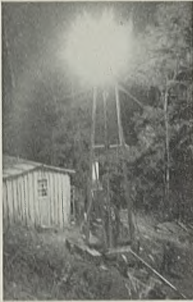
Gas estimated at 150 c.f.m. is burning at the top of this core drillhole, one of four which have reduced the gas content in an underlying mine section from 1.5 to 0.3 per cent.
