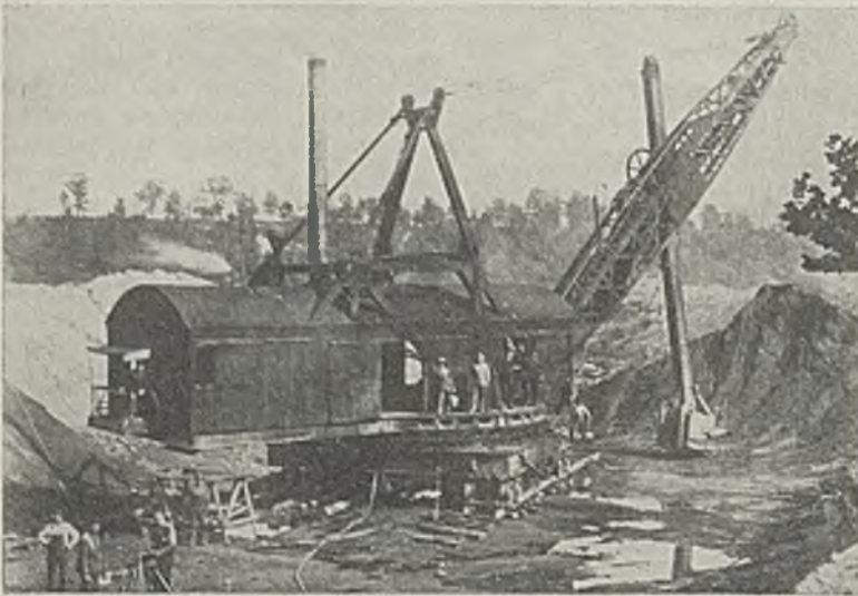
1911 — "World's largest" shovel digs in with its 3-cu.yd. dipper at Danville pit
