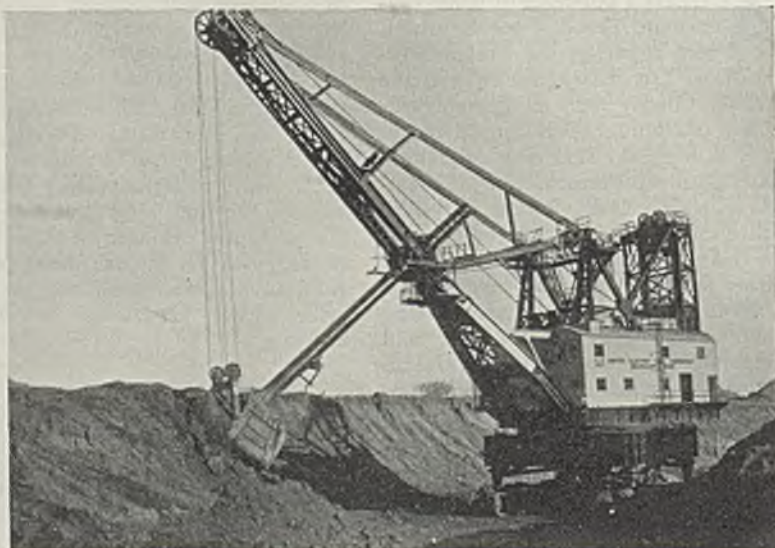
Electric shovel with 30-cu.yd. dipper at work stripping off the overburden
