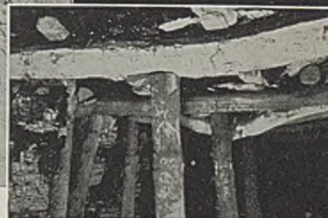
Broken bars in air-course replaced by K-R pressure treated bars.
