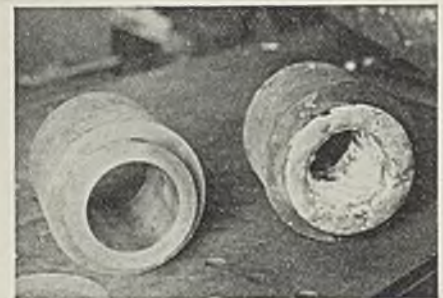
"Bronzed-up" new cage rollers last twice as long as solid cast-steel rollers. Here is a welded and a finished roller on the welding bench, Zeigler No. 2 mine.
