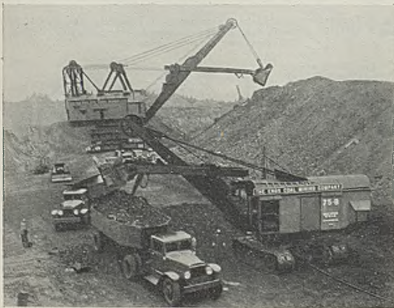
View of the No. 2 pit at Enos, showing stripping, loading, haulage and auxiliary operations.
