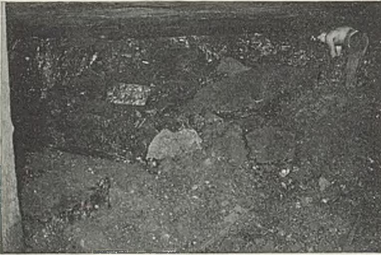
Left half of a typical room in Nokomis mine after the face is shot down. The large lumps are derived from the top round of holes
