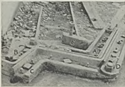
Fig. 2—Second and final bend completed to reshape iron
