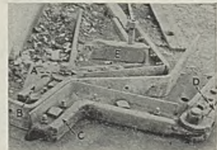
Fig. 1—Iron in place ready for rebending
