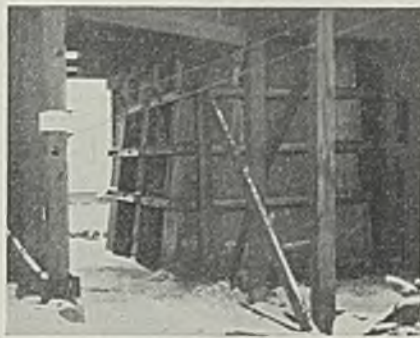
How the pier looked after reinforcing was completed
