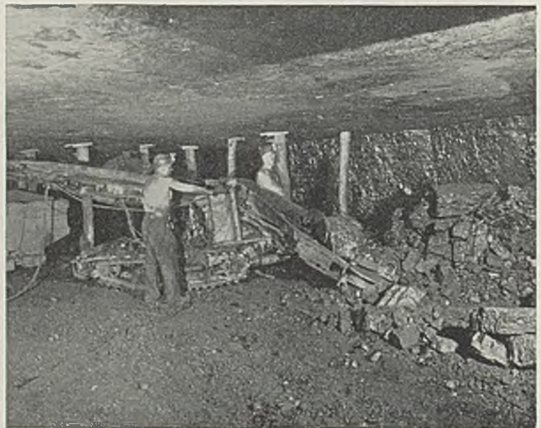
Loading machine moving into the coal shown in the illustration above
