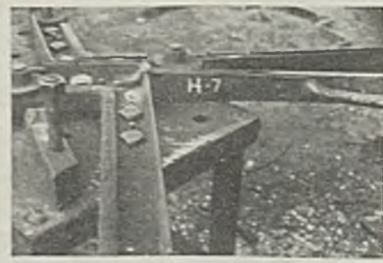
Fig. 18—Showing use of the stop gage (Fig. 19) to position the iron for bending
