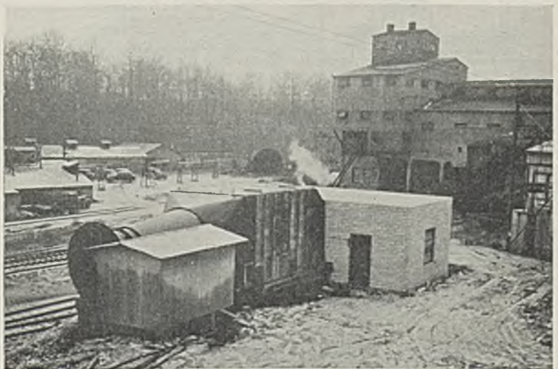
Talleydale ventilating and air-conditioning units. At the left is the fan with the motor house in front of it. Next to the fan is the air conditioner, which connects into the housing over the air shaft. At the right is the room housing the service pumps and electrical apparatus and controls
