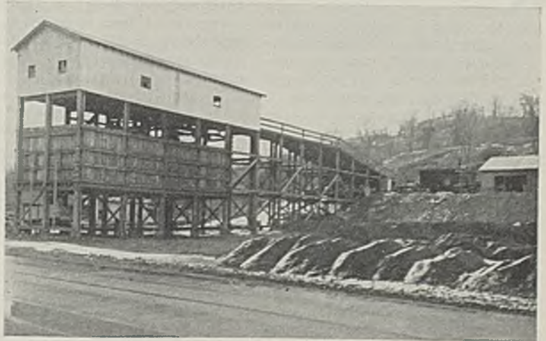
Below the tippie, which has a shaker screen, are four 110-ton bins. Slack in the right foreground was thus stored because it would not sell at the minimum prices set by the code.
