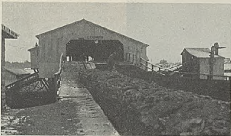
A 5,965-ft. rope haul delivers 28-car trips to this point, where a loaded trip puller completes the haul into the tipple.
