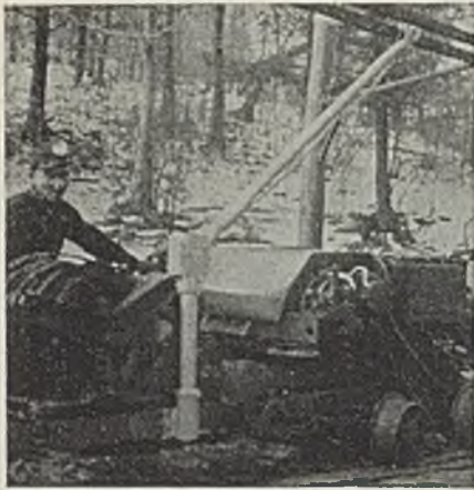
Pole in place on the machine truck
