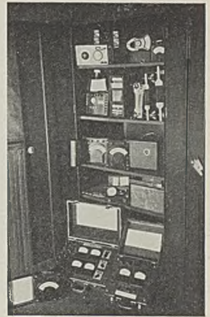
Isabella metering equipment. A graphic watt-hour meter was in use when this photo was taken and consequently is not shown.
