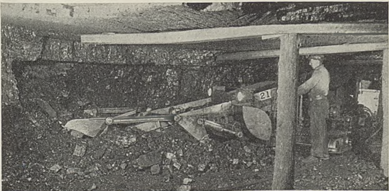
Loading machine starting a cut-through in a pillar at Isabella.
