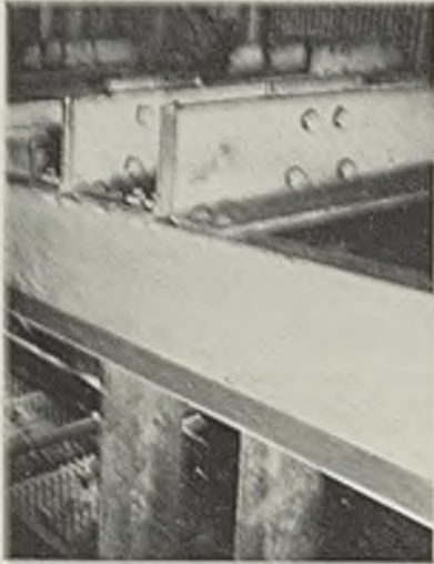
Rounded corners on these hanger supports reduce likelihood of breaking the arms.
