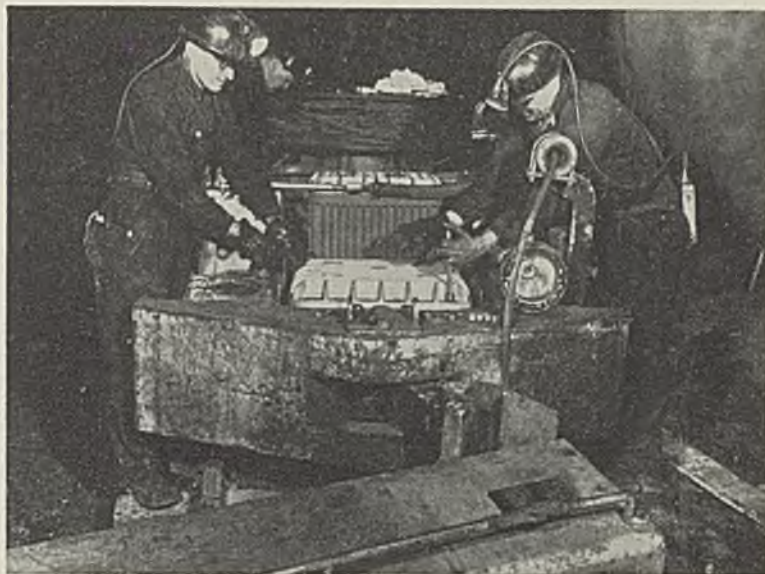
Regular equipment inspections are the rule at Isabella. Here one of the new 8-ton cable-reel locomotives is receiving its regular weekly check.
