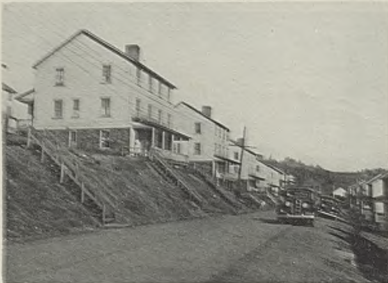
Looking down the main street in Isabella. House renovation included asbestos-shingle sidings, new steps, rebuilding porches, etc.
