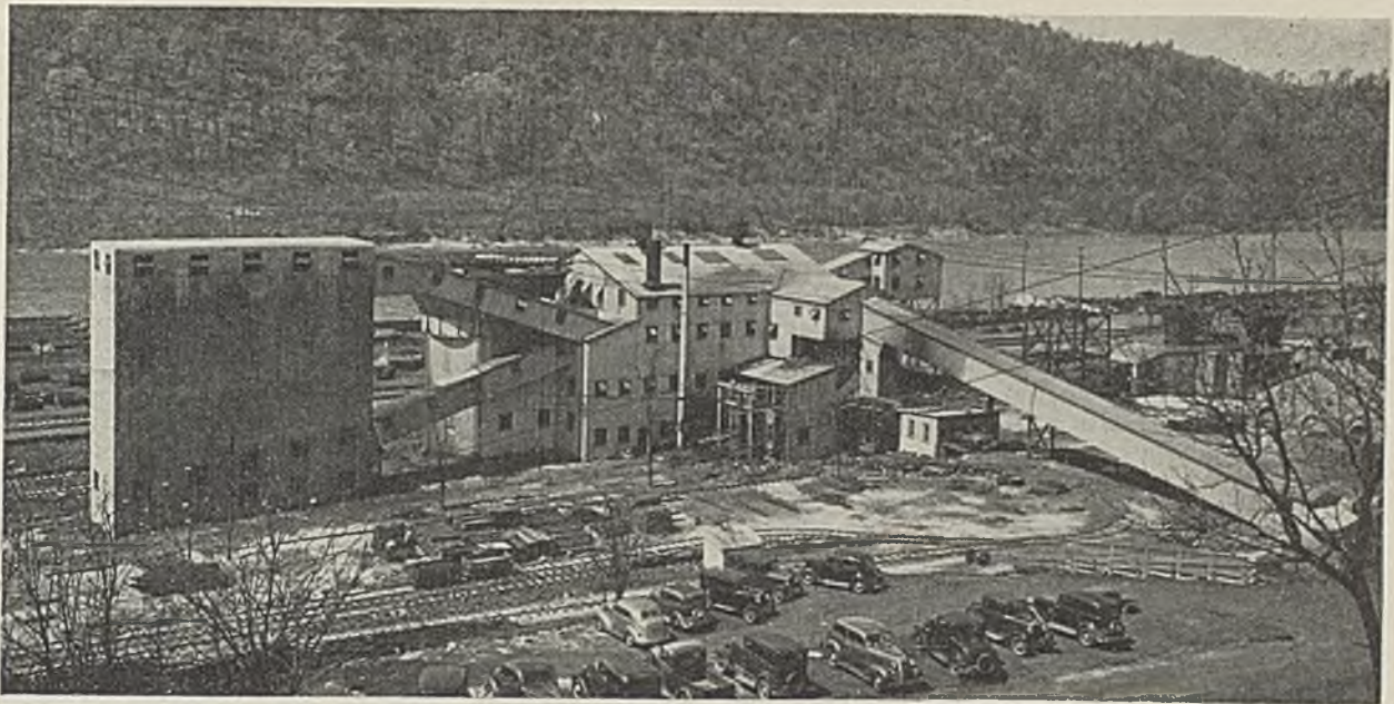
Isabella metallurgical-coal preparation plant. The blending plant is at the left, with the slope-conveyor gallery at the right.
