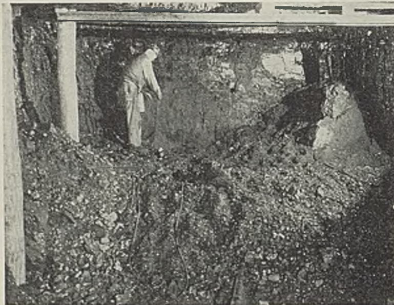
Wiring up shots in a rib place, showing use of the 15-ft. auxiliary cables which are attached to the detonator wires.
