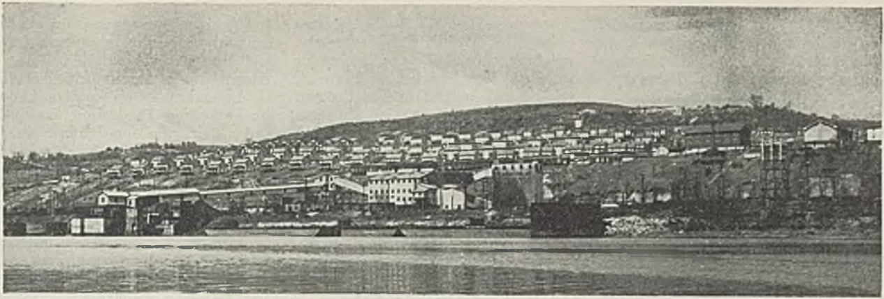
Isabella surface plant and town lie along the northern bank of the Monongahela River
