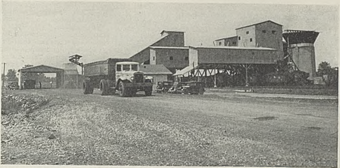
This plant prepares coal from Nos. 23 and 24 mines on separate days or separate shifts. The drying plant is behind the settling cone
