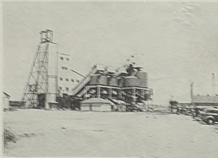
New Centennial preparation plant. The screening section is built onto the shaft headframe and is connected with the truck-loading bins by inclined conveyors. At the extreme right is the tail tower of the aerial tramway.
