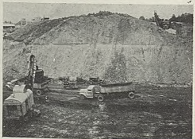
View of the Maumee No. 23 pit, with the stripping shovel around the turn at the right
