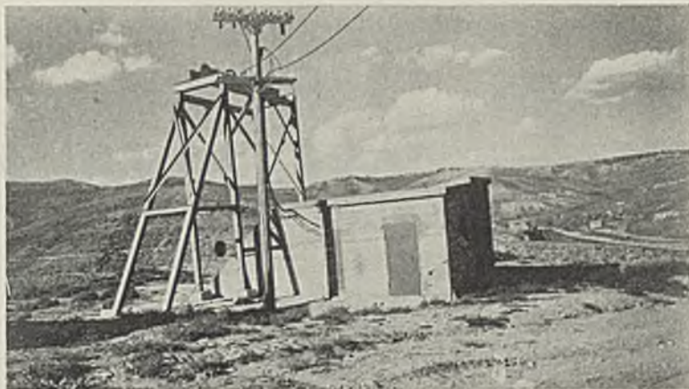
Fan at No. 7 shaft. Note rolling terrain.
