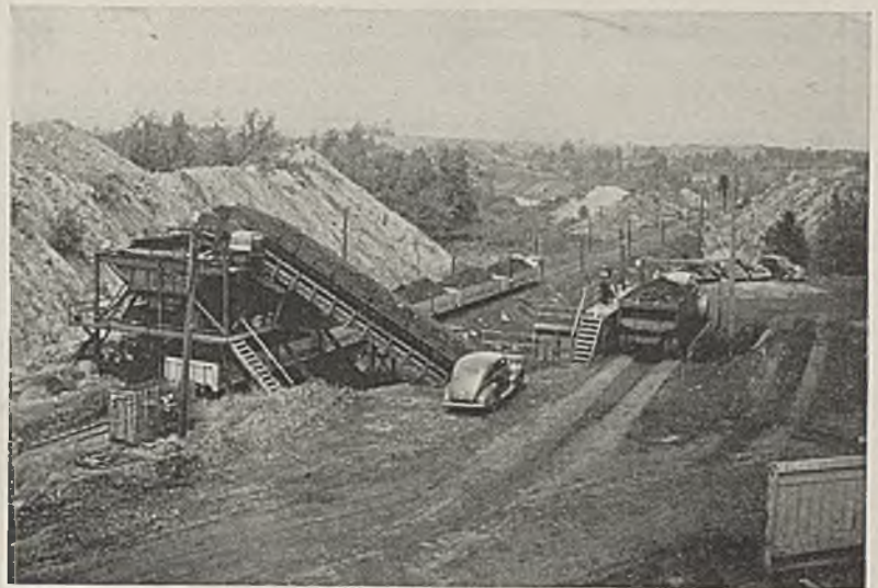
Enos field transfer station, with one of the electric trains loaded ready for its 4½-mile trip to the preparation plant.
