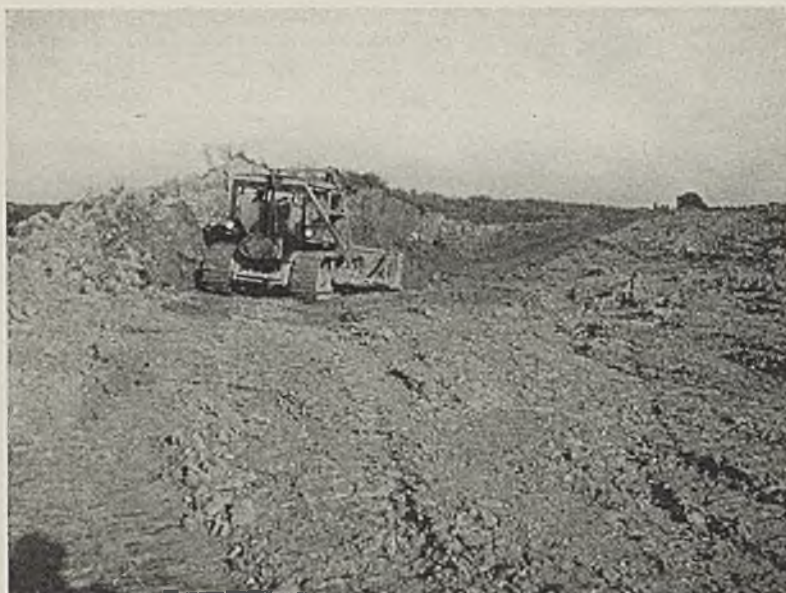
Spreading slide material on the bank at Bobolink mine.
