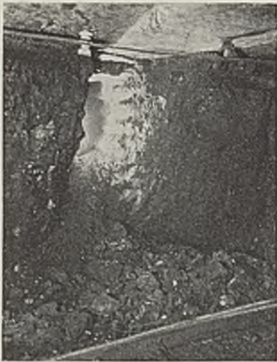
Result of a shot to make a rib hitching for a seal in Kings Station mine.
