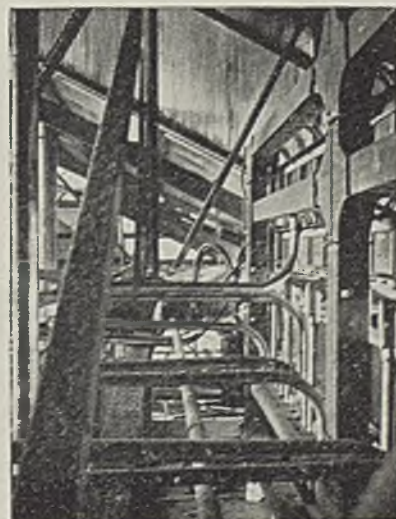
Right: square duct protects wire groups between rigid and flexible conduits.
