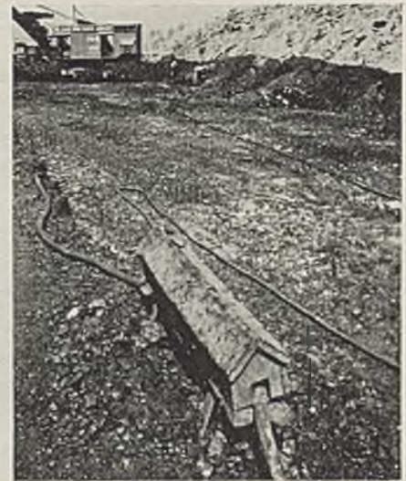
Connector box serving a 5-yd. loader at Enos.
