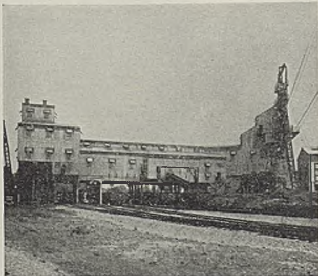
All coal is washed in this preparation plant at Talleydale mine.
