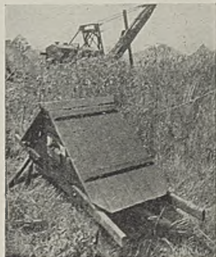
Portable interlocked oil switch serving the stripping shovel at Ayrshire.
