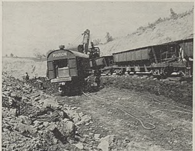
Loading 44-ton standard-gage cars in one of the Ayrshire pits.
