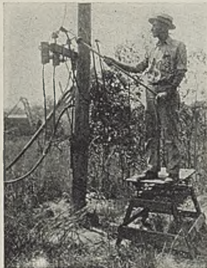
Here the "conductor" is in the center of a series of insulators.
