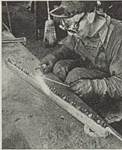
Patented renewable bits are tipped at Saxton.
