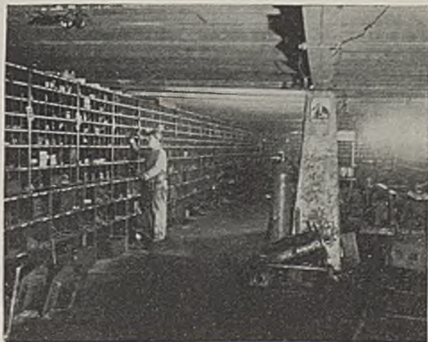
Steel bins occupy 196 ft. of wall space in the underground central supply room at Kings Station.
