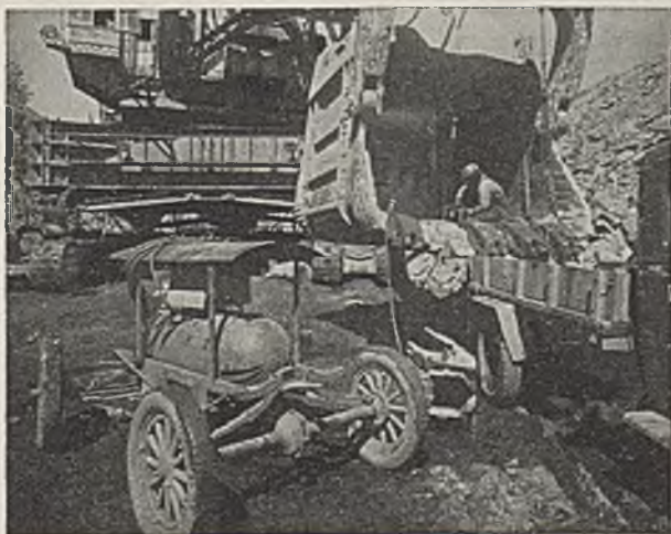
Arc-welding the 30-yd. dipper at Binkley's Bobolink strip mine.
