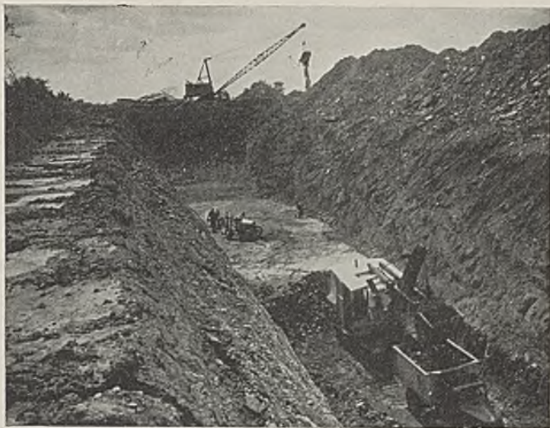
As is usual in most dragline operations, all the coal is being loaded in the Beech Coal Co. pit.
