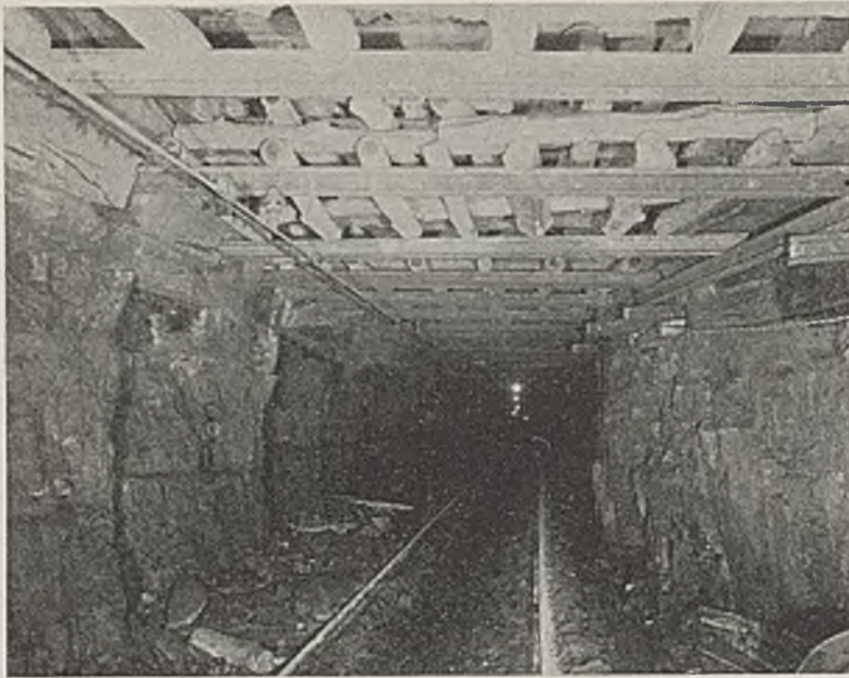
Hitch-drill timbering in a reopened haulage road at Miami No. 10, showing the use of pins and stringers on the chain-pillar side (right) and single holes on the barrier-pillar side (left). The left side was widened 3 ft. after the crossbars and lagging were installed.
