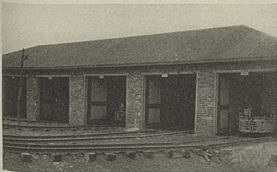
Battery Equipment Barn, Louise Mine
