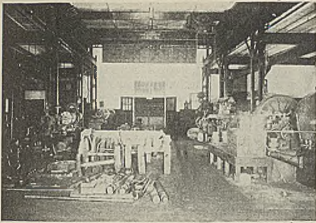
Machine Tool End of the Center Bay
