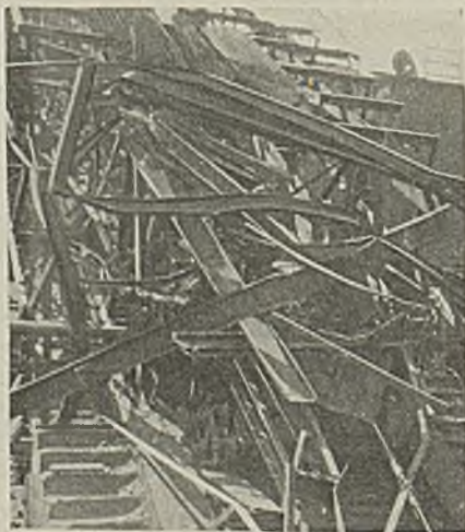
Twisted Mass of Steel at Ground Landing
