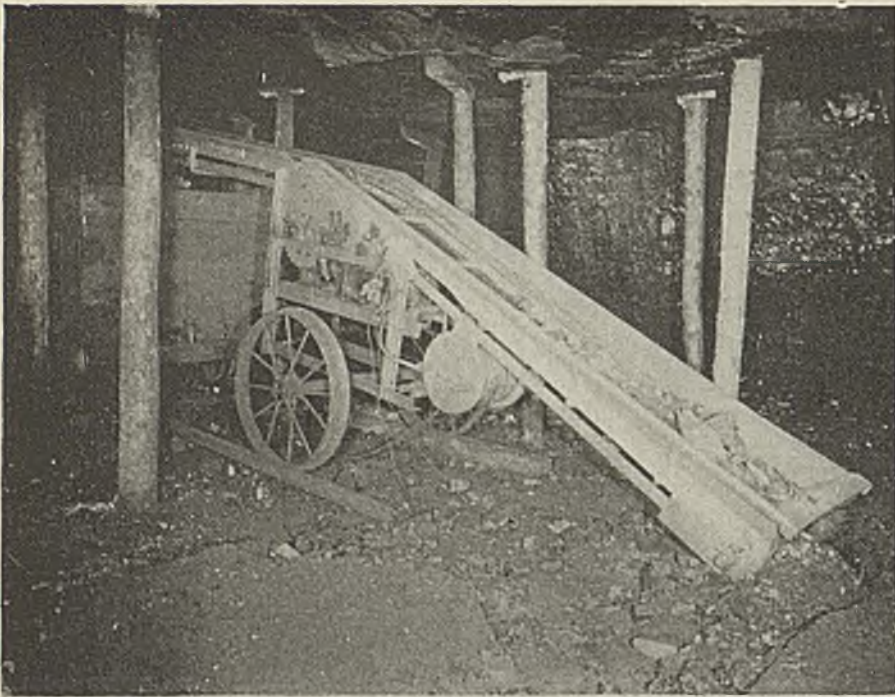
Light Weight Makes It Practicable to Take This Conveyor Off the Track Onto the Bottom Coal
