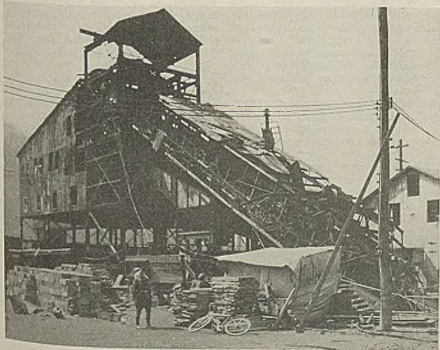
Tipple Damage by Force and Flame
