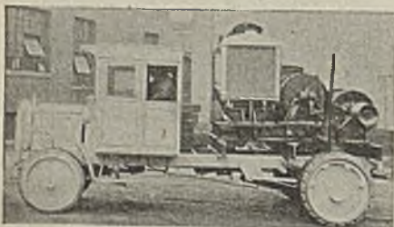
Ready for Dragline Operation
