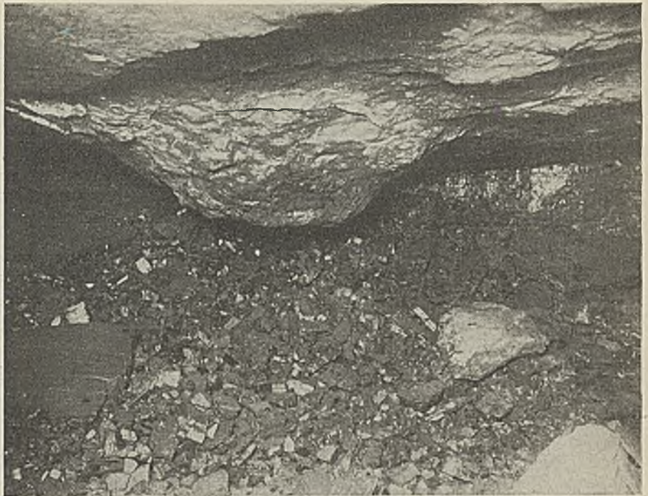
This Horseback in 7½ Ft. of Coal Comes Down to Within 4½ Ft. of the Rail
