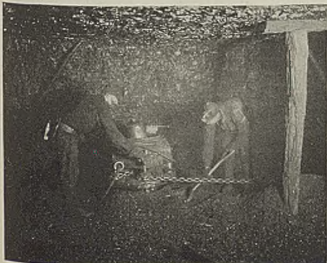
Failure to Use Water on the Cutting Chain Causes the Air to Be Filled with Minute Particles of Coal Dust, Likely to Forward an Explosion
