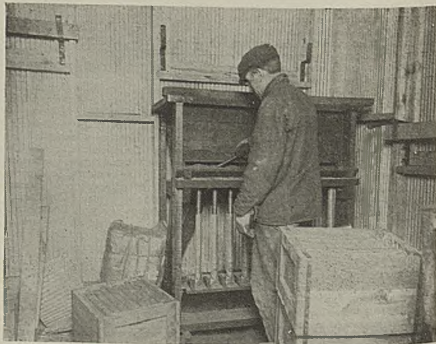
Stirring the Sand Into the Loading Tubes
