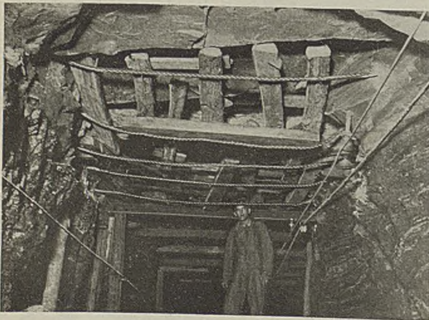
After Two Years These Ropes Continue to Hold Badly Fractured Roof
