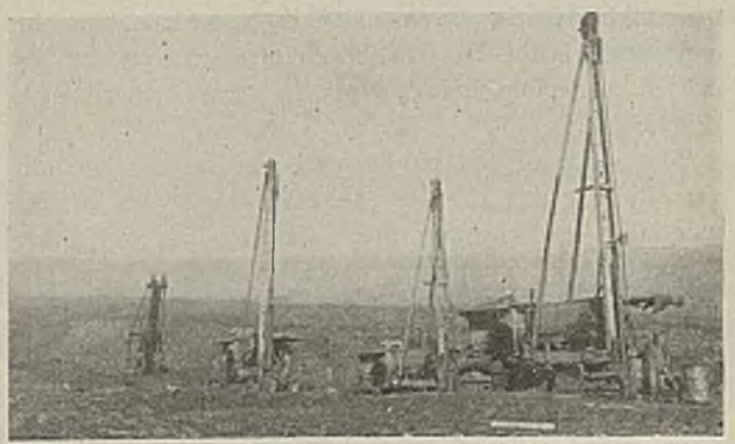
Caterpillar Mountings Take These Electric Drilling Machines Over Rough, Muddy Ground
