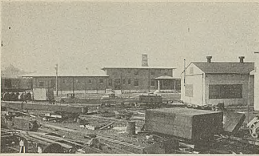
Left to Right: Machine Shop, Office and Warehouse
