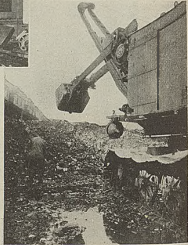
Twelve Yards or More at a Bite Scooping Up 5½ Ft. of Coal
