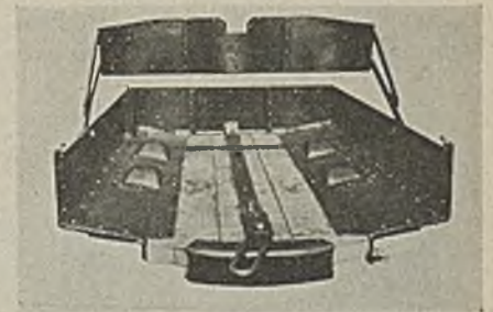
Fig. 13—New Construction for Lowness and Large Capacity
