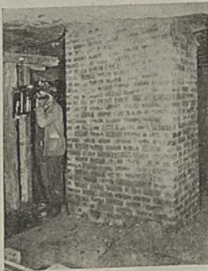
Brick Pillar Protecting Terminal Of a 6-Pair Branch Cable
