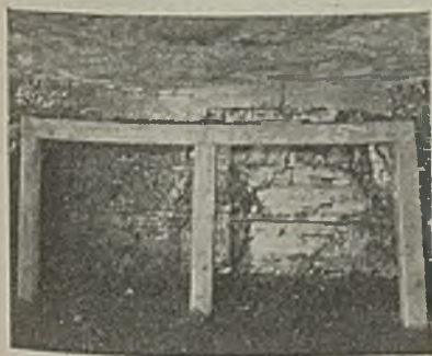
Where a Timber Set Is Needed
