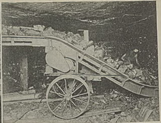
Conveyor on Balled Rails in Franklin Mine
