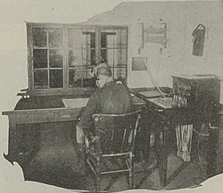
Tending the Switchboard is Part of the Dispatcher's Job
