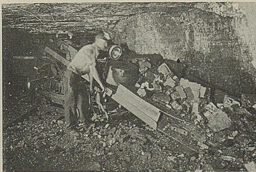
Fig. 8—Loading Out the Second Cut in a Breakthrough
