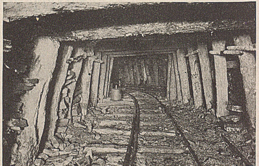
Guard Rail on a Plane Branch
