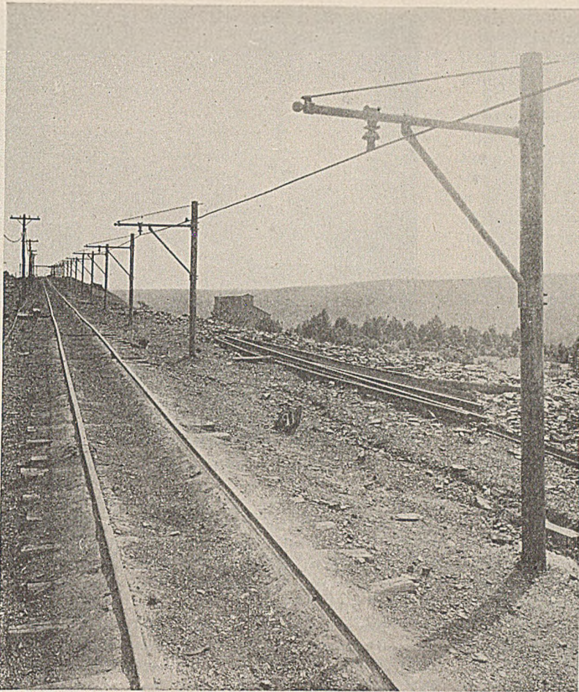
Rugged Trolley-Line Construction at Clinton Colliery
