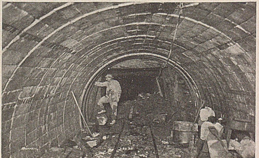
Fig. 2—Intrados of Completed Arch
