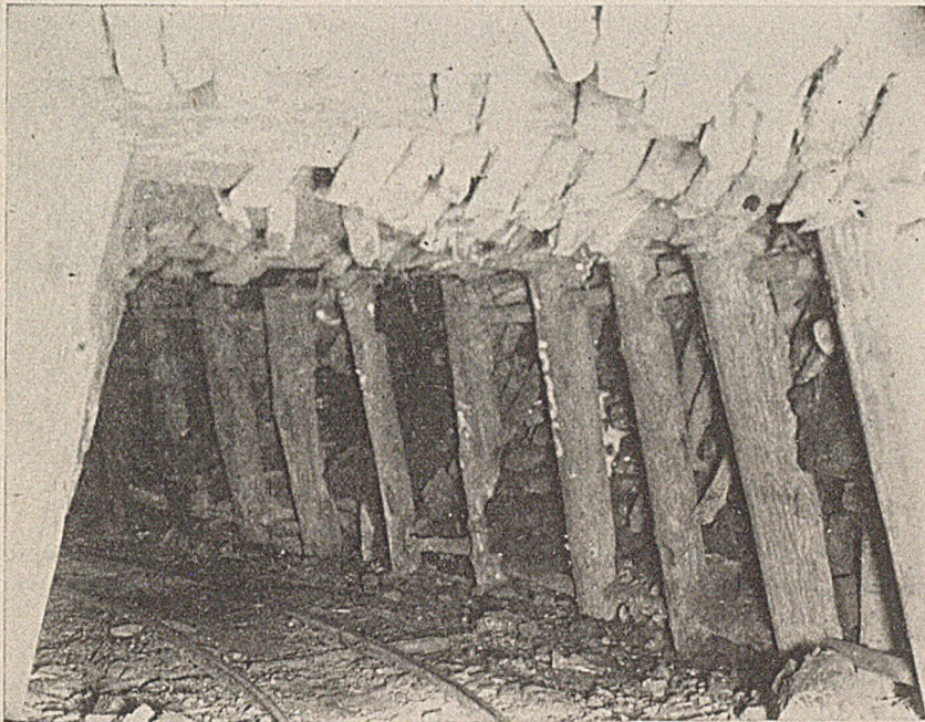
Forepolling in Loose Ground
